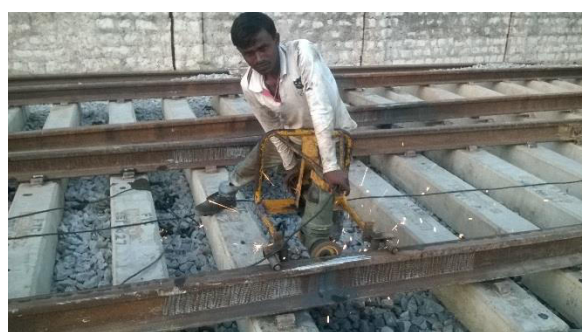
Workers seen without PPE at track welding in HT-1
