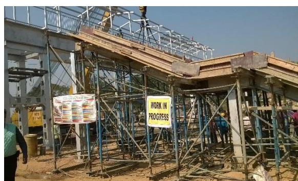
Launching work for FOB at Godbhaga Railway Station in ST-2
