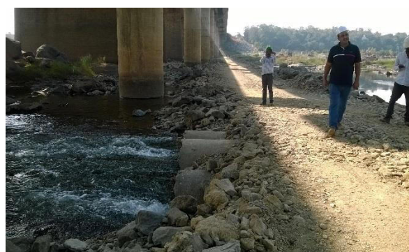
Hume pipes provided for water flow under approach road at Hirapur bridge in ST-1
