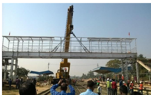
Launching work for FOB at Godbhaga Railway Station in ST-2
