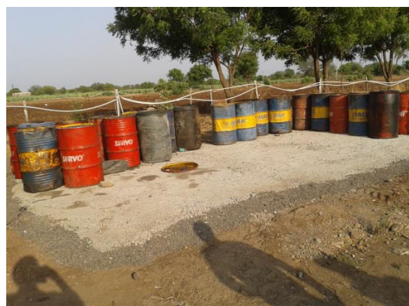
Petroleum products stored on impervious platform at DG-2
