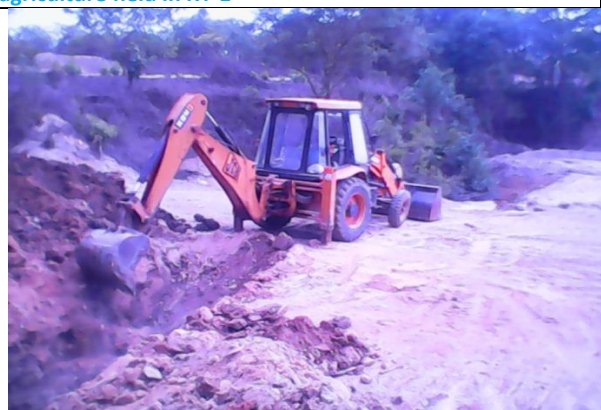
Clearing of blocked water way at bridge No. 113 (Ch. 543/700) in HT-3
