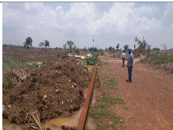
Debris lying along the rail bed in RT-3 near ch: 32 require removal
