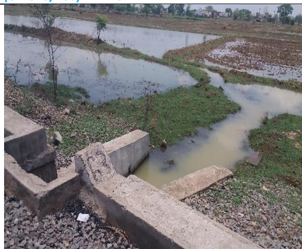
Flooding of surrounding area due to blockage of vent at Bridge No.63 ch.32 in RT-3.
