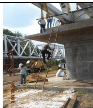
Safe working platform required at Sukhtal (Bridge No. 331) in ST-1
