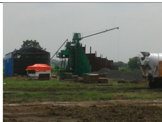
Batching plant at Sawalgi in DG-2
