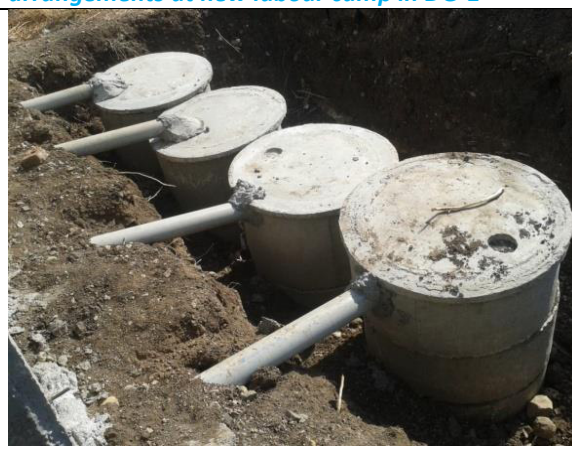
Toilet units with septic tank under construction at new labour camp in DG-1
