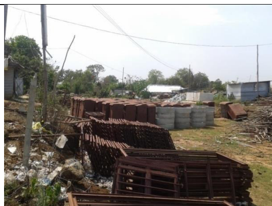
Stacked construction materials blocking the natural waterway at Alnawar camp site in HT-3, require shifting
