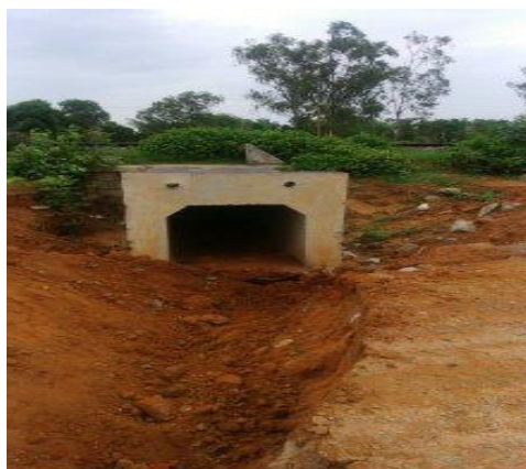
Vent clearance at bridge No. 99 in ST-2
