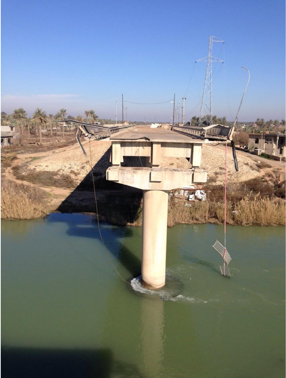
Figure 9: Damaged span in the small bridge (2)
