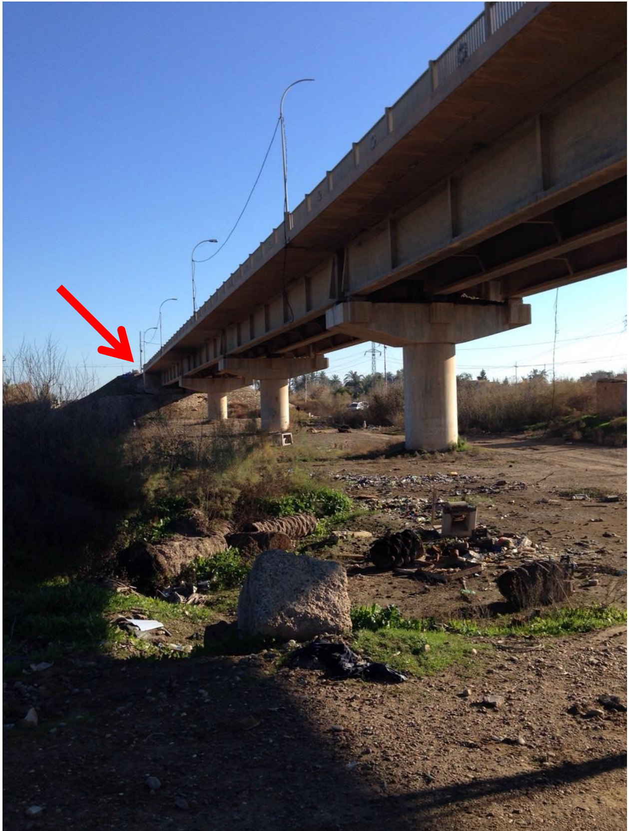
Figure 7: Damaged span in the big bridge
