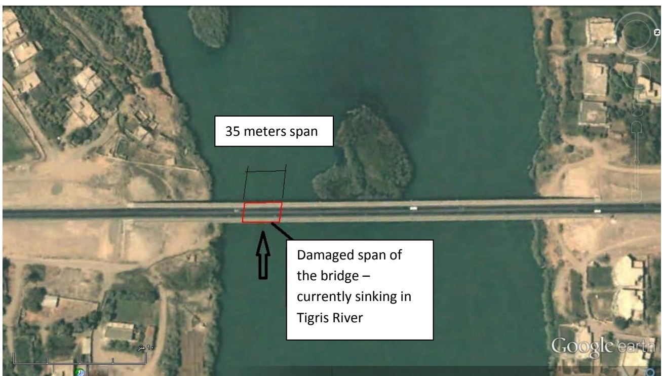
Figure 5: aerial photo of Al-Dhuluiya big bridge
