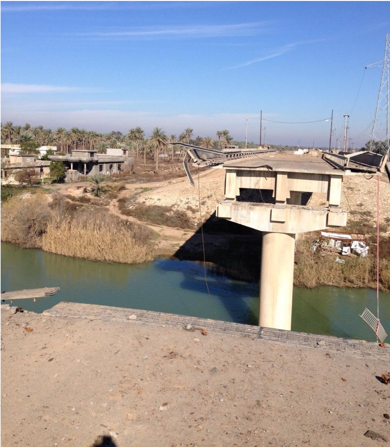
Figure 8: Damaged span in the small bridge (1)
