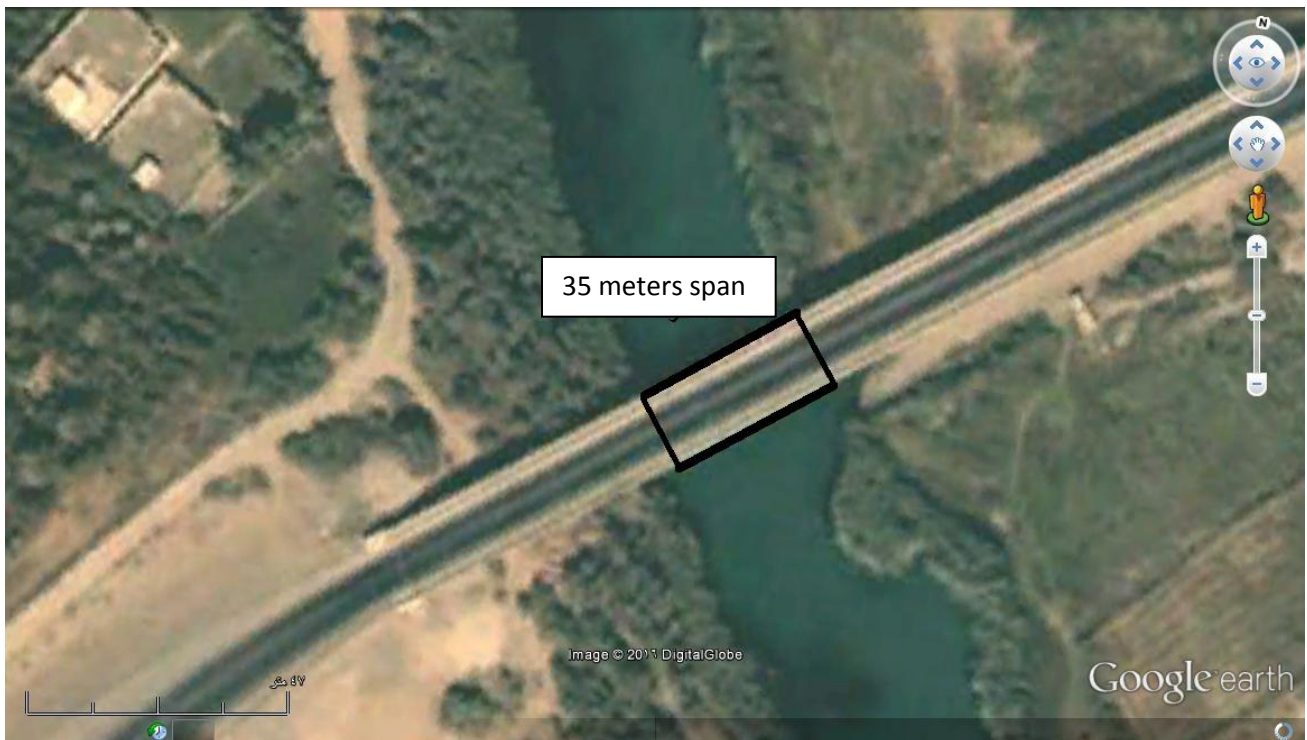
Figure 4: aerial photo of Al-Dhuluiya small bridge
