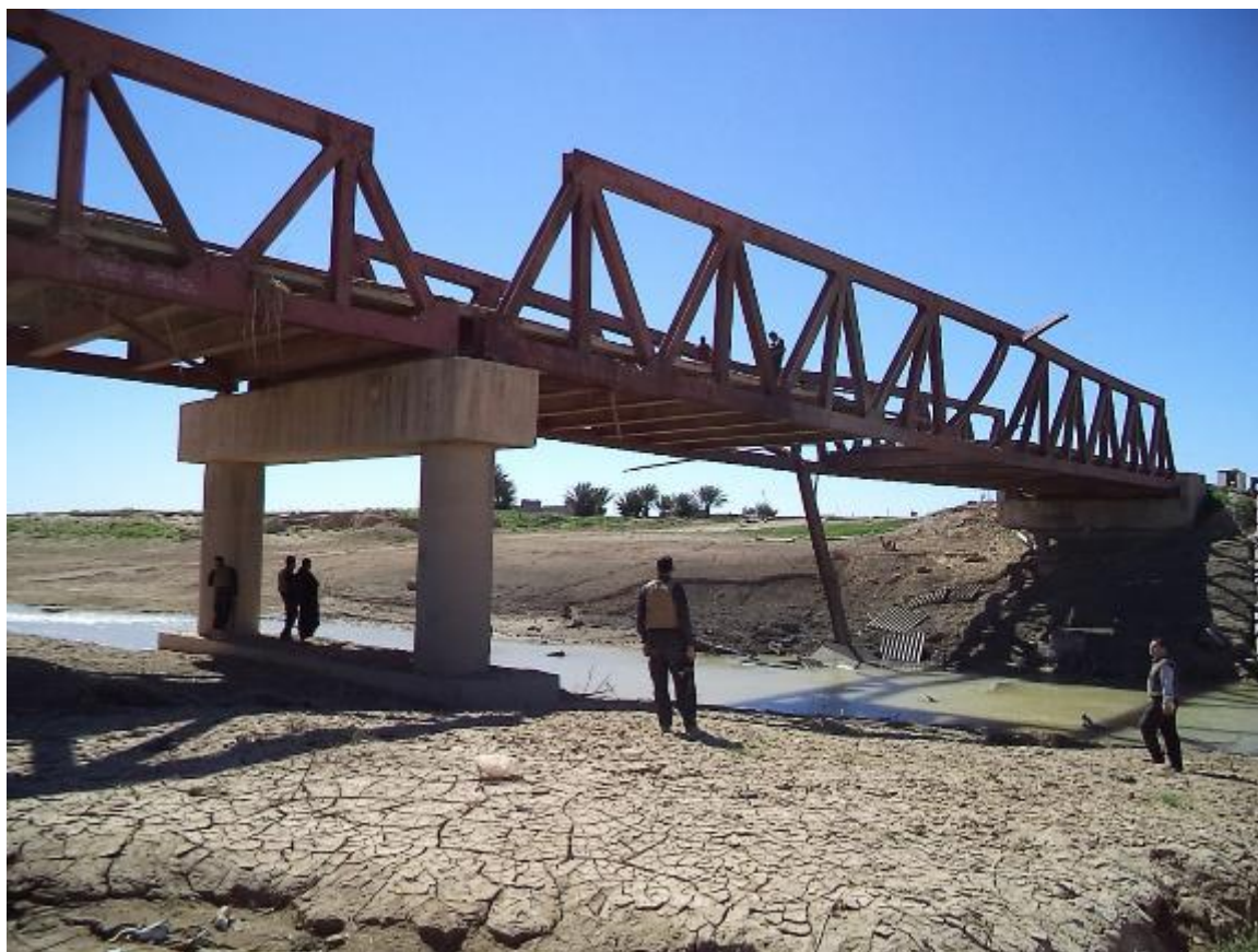
Figure 3: General View of the steel bridge
