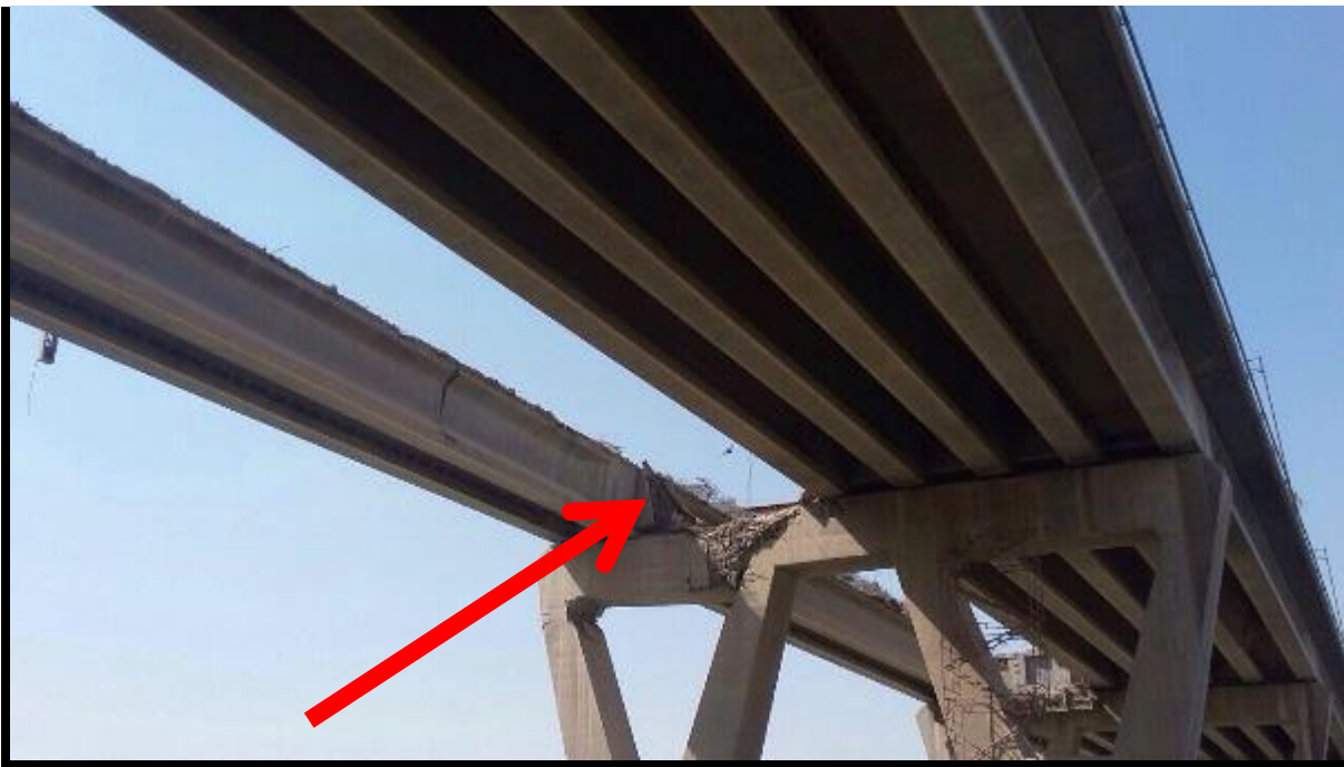
Figure 7: Damaged span in Bridge
