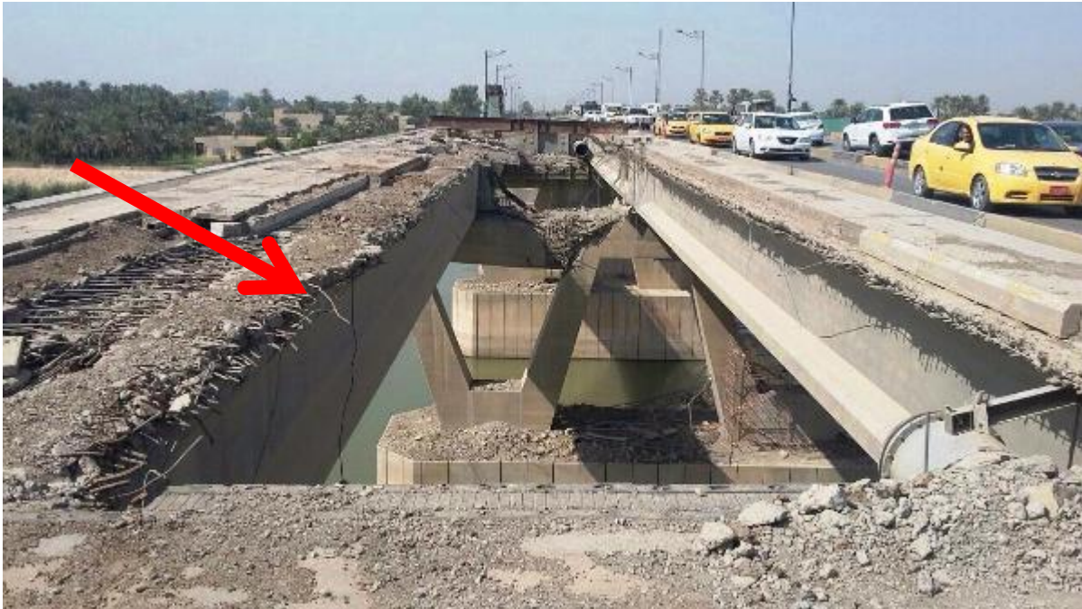
Figure 6: Damaged span in the Bridge
