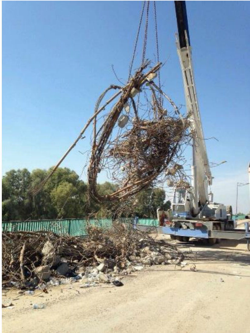
Figure 8: Damaged span in the Bridge being removed clear the way for traffic
