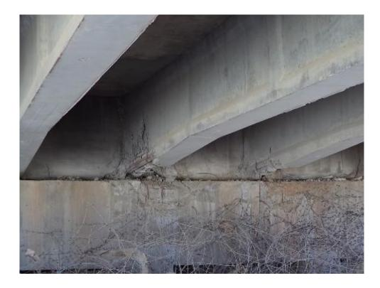
Figure 8: A zoomed view on the damages of Bridge (4) on Imam Way
