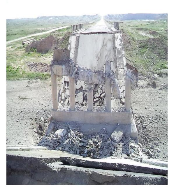
Figure 11: Span completely demolished on Bridge (7)
