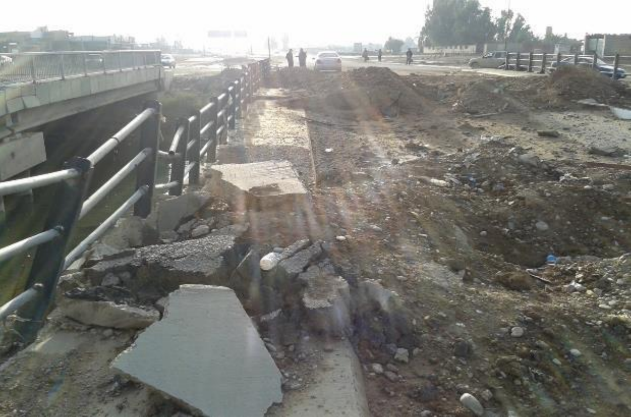
Figure 5: Damaged and un-trafficable span of the old bridge
