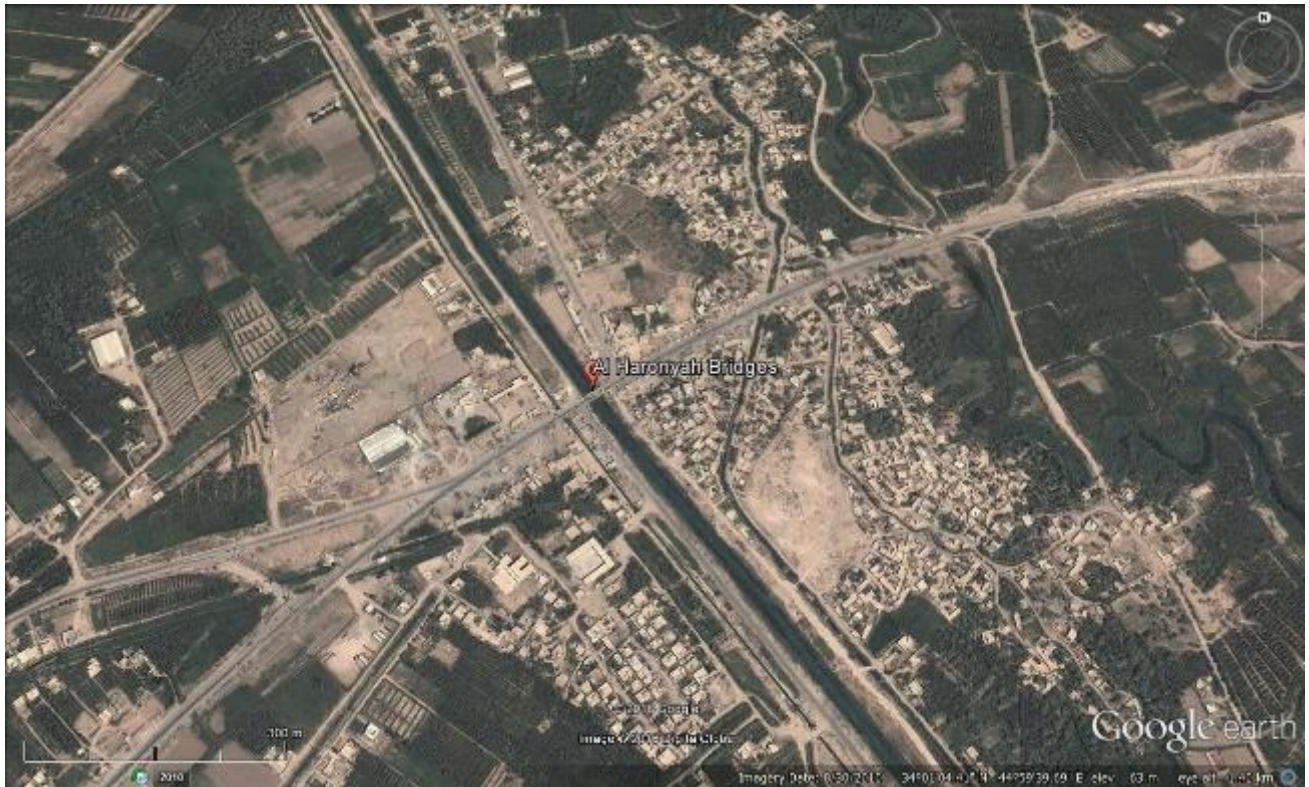
Figure 3: Land use around Al-Haronyah Bridges (Google Earth)
