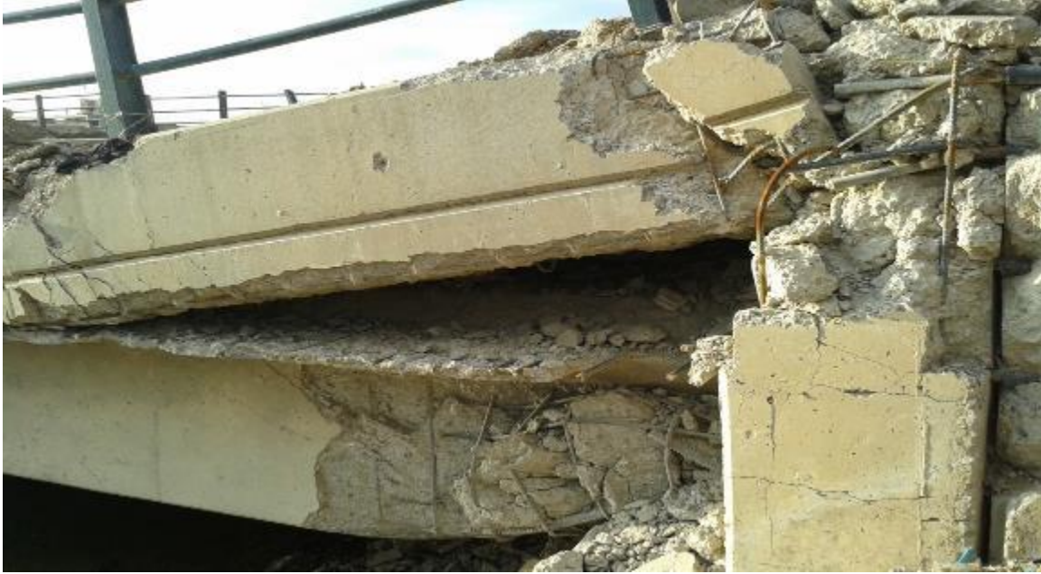
Figure 5: Damaged span in the old Bridge
