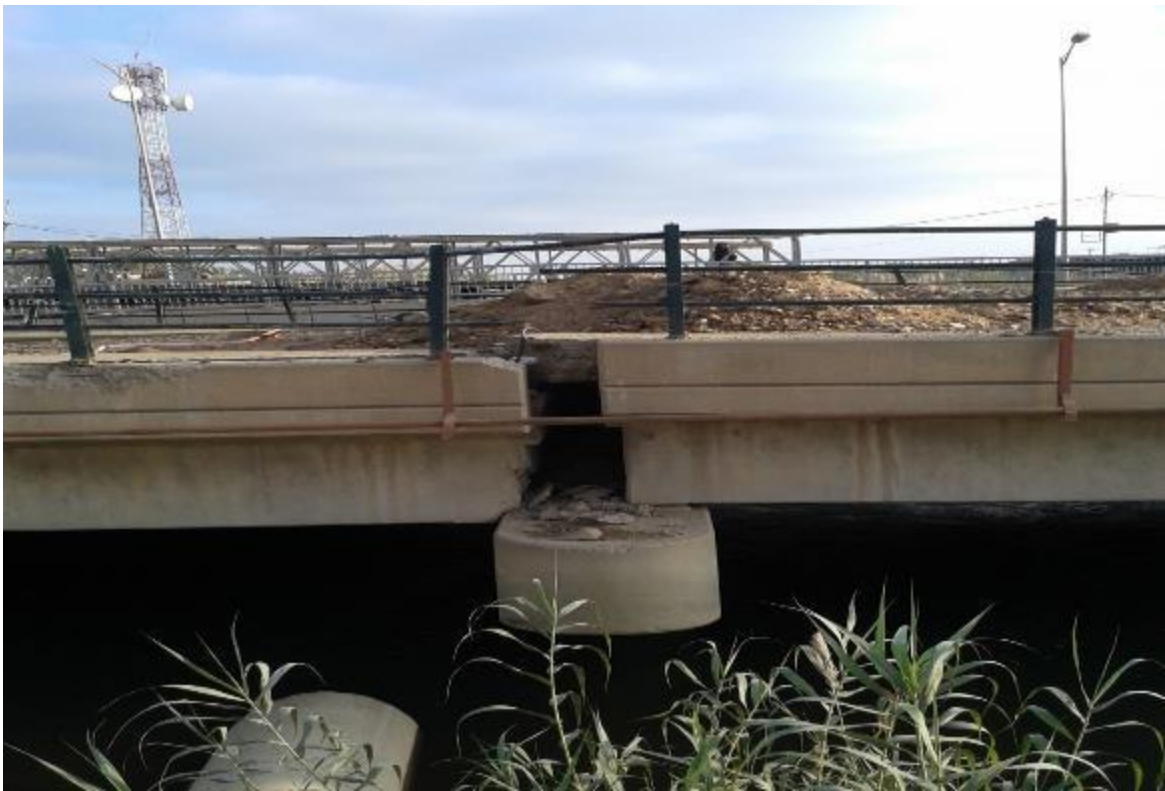
Figure 8: Damages in the old bridge
