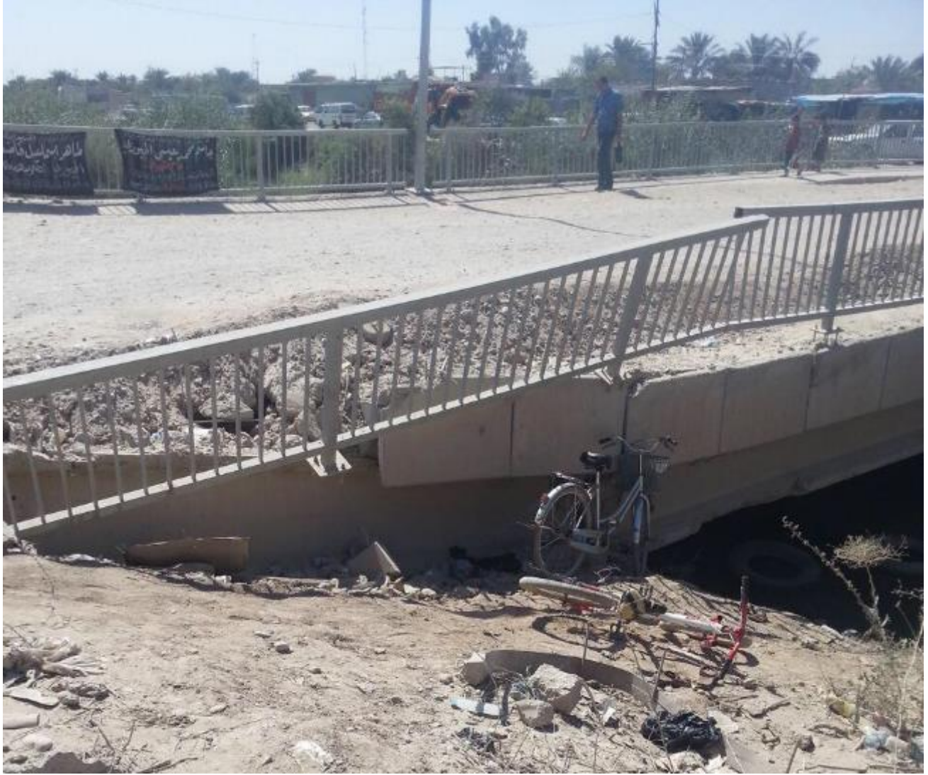
Figure 6: Side view of damaged Haronyah new bridge
