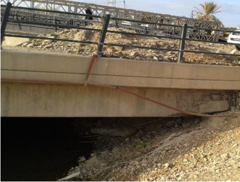
Figure 7: Side view of the damaged span of the old Bridge
