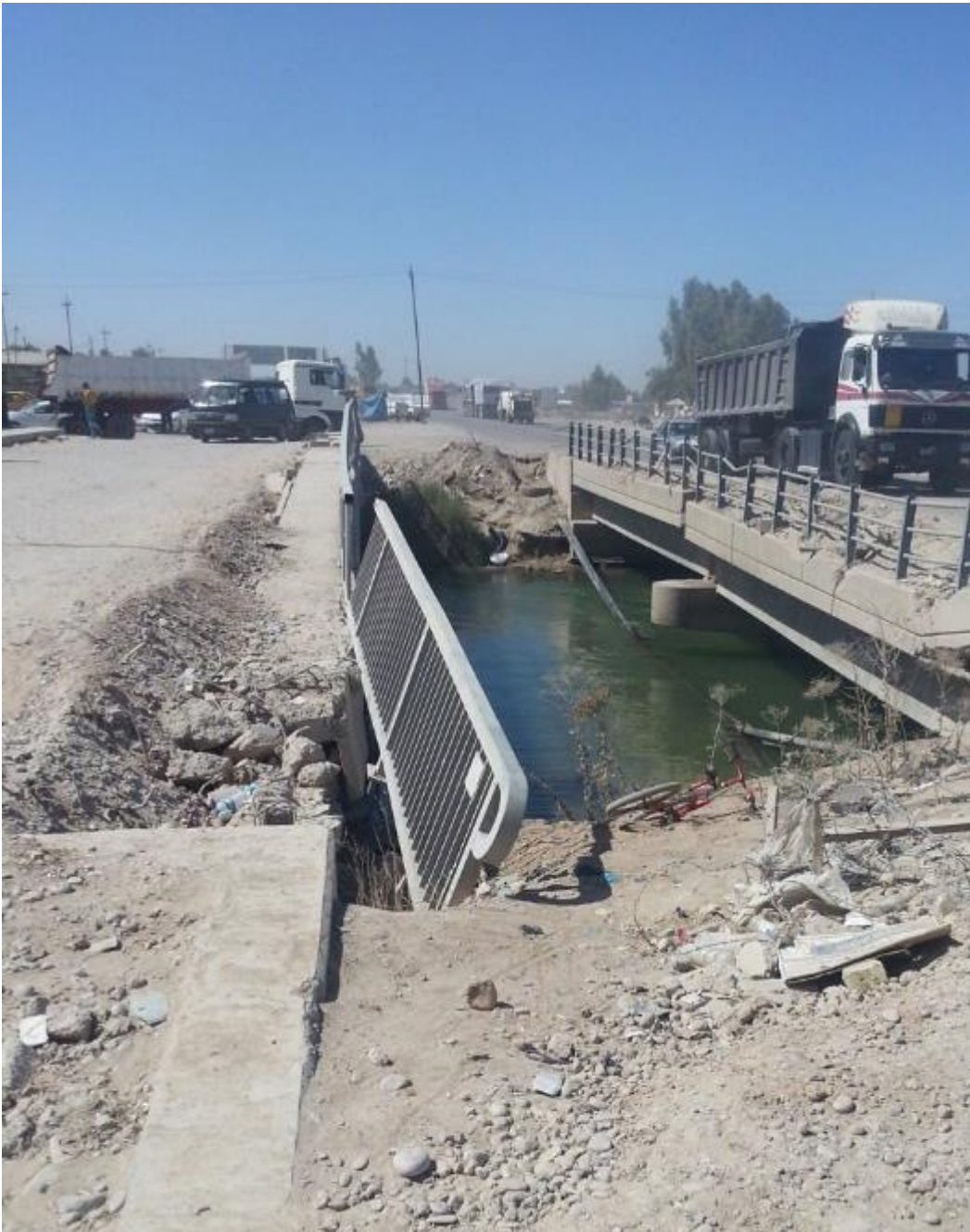
Figure 4: Photo showing Al Haronyah old and new bridges
