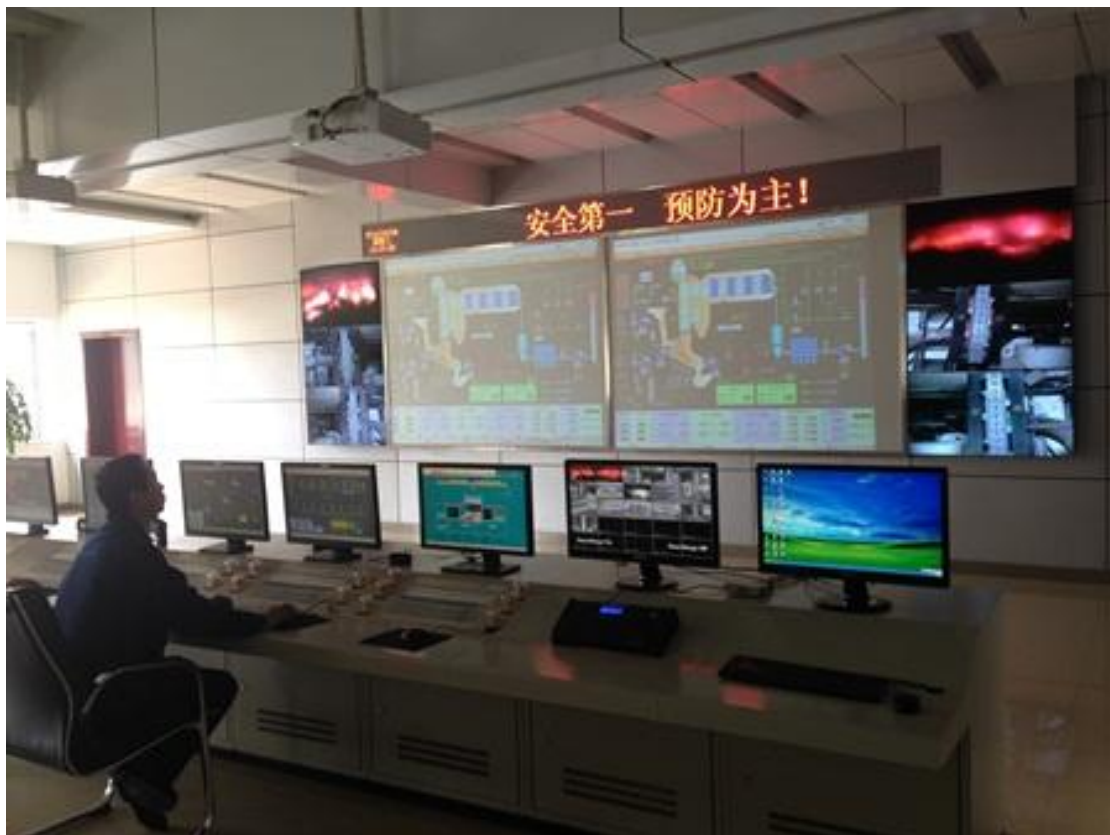
Figure 5-3 Konggang Incinerator's Central Control Room
