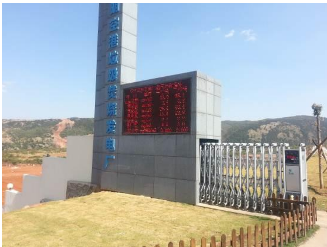
Figure 8-3 Emission information disclosure at the gate of Konggang incineration plant
