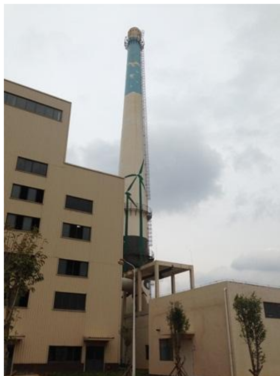
Figure 6-2 Konggang Incinerator Stack and Online Monitoring Sampling Spot
