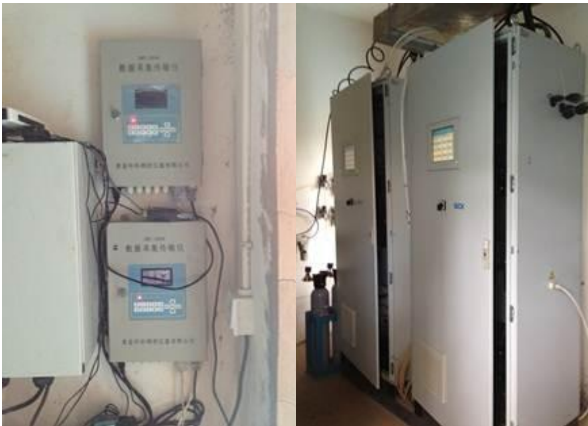
Figure 6-3 Konggang Air Emission Online Monitoring and Data Transmitter
