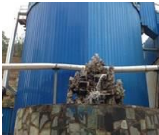
Treated wastewater reused at fountain in Xishan
