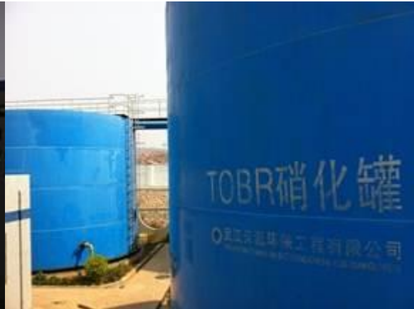
Dongjiao aerobic nitrification tank
