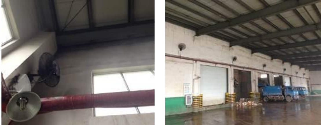
Figure 5-1 Spraying of plant extract liquid through fans at offloading area (Xishan Incinerator)
