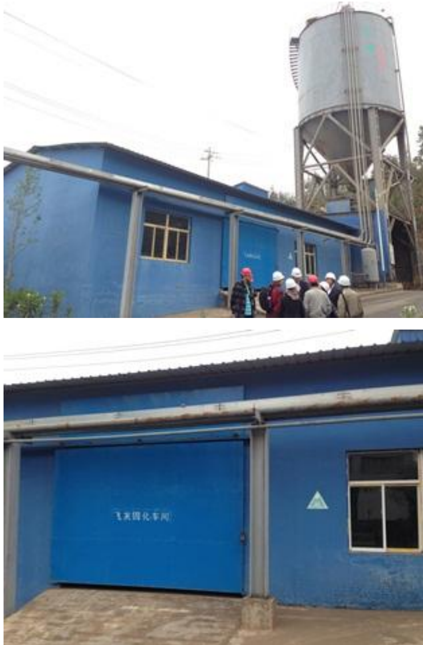
Figure 6-4 Fly Ash Stabilization Workshop in Xishan Incinerator
