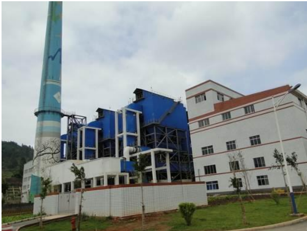
Figure 5-7 Flue Gas Treatment and Stack, Xishan Incinerator
