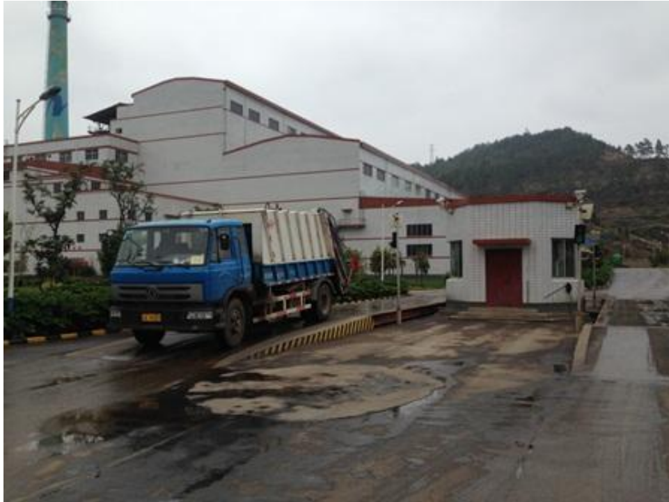
Figure 5-3 MSW Weighting in Xishan Incinerator
