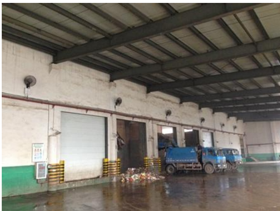
Figure 5-5 Odor Removal Through Fan in MSW Offloading Area, Xishan
