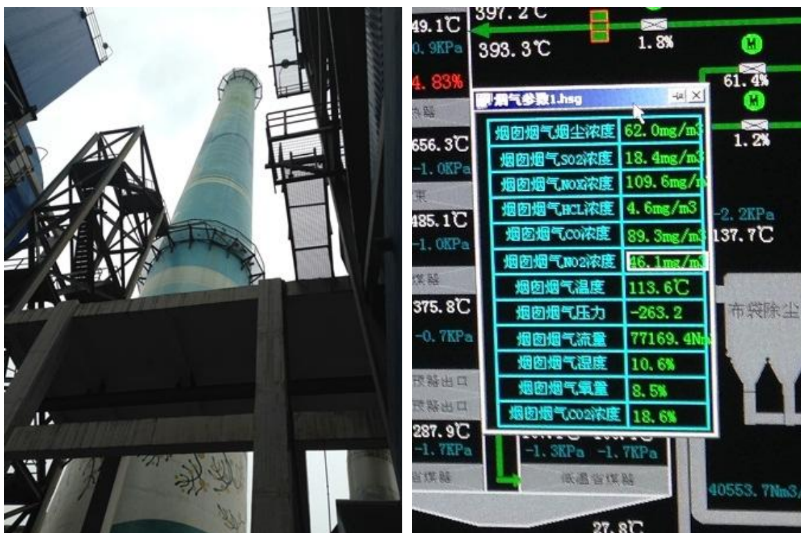
Online monitoring Spot in the middle of Stack Online monitoring data available at central control room
