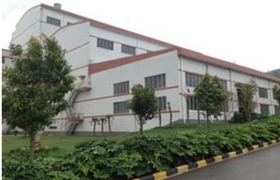
Figure 5-4 Waste Pretreatment Workshop in Xishan Incinerator
