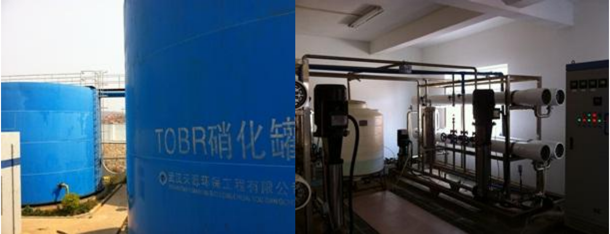
Figure 5-7 Dongjiao Leachate Treatment System
