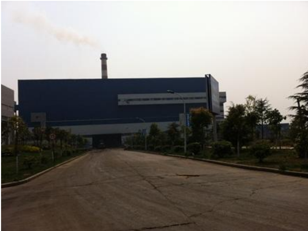
Figure 5-4 Dongjiao Incinerator's Offloading Workshop
