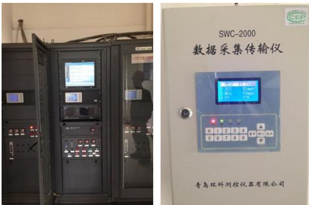
Figure 6-3 Dongjiao Online Monitoring and Data Transmitter
