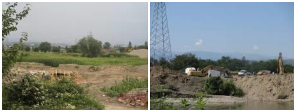
Figure 4: Photos of Activities at Project Location
