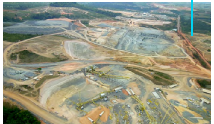
Belo Monte Dam construction 2013.
