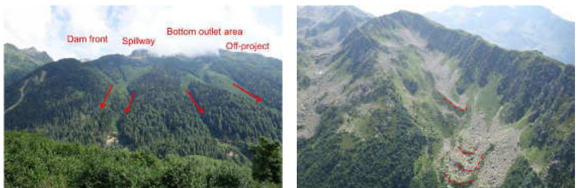
Debris flow/avalanche channels on the left slope above the dam (left) and uphill area of the rightmost channel (right).
