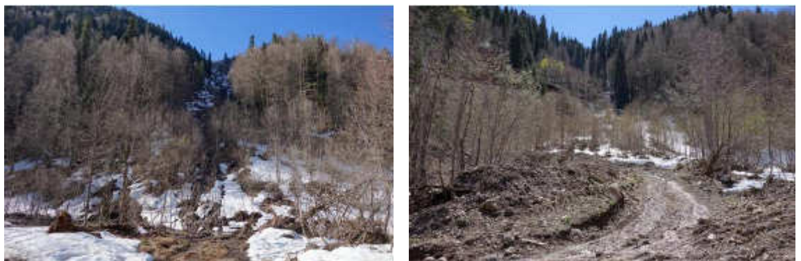
Alluvial/debris fans with possible debris flow and snow avalanche activity which point towards the upstream face of the dam (left) and the initial and middle/final part of the surface spillway (right).
