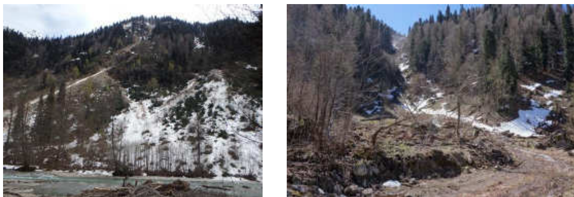
The intake portal of the Bottom outlet tunnel is located at the foot of the snow-covered debris fan on the right of the photograph (left). The alluvial/debris fan with snow avalanche activity which points towards the area of the exit portal of the Bottom outlet tunnel (right).
