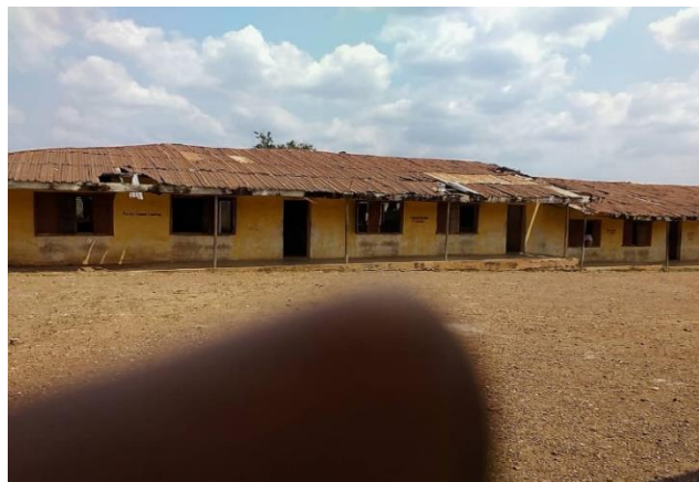
Plate 5: Bent and falling roof on building
