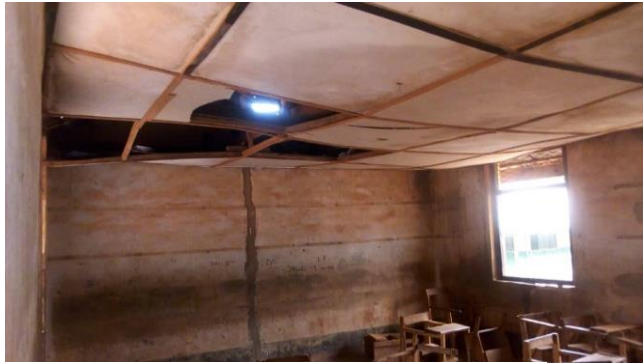
Plate 7: Asbestos ceiling
