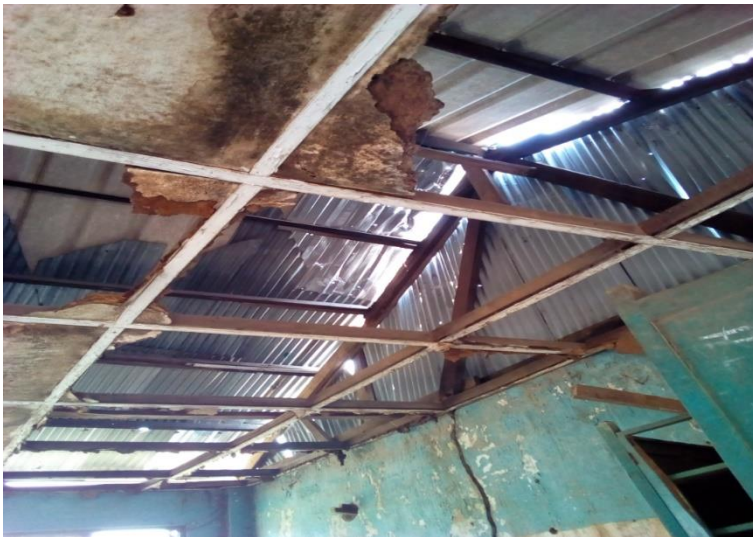
Plate 20: Damaged and rotting asbestos ceiling, Cracks on the walls
