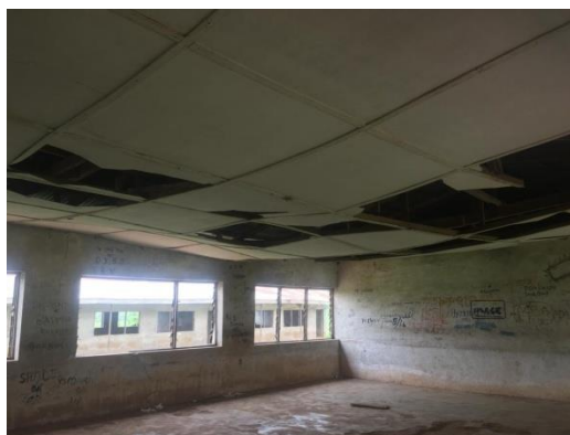
Plate 12: Asbestos ceiling
