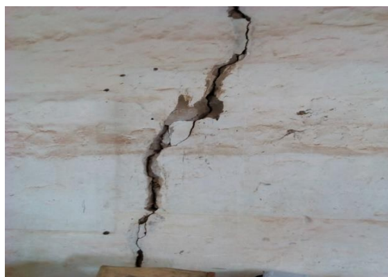
Plate 18: Figure 10: Cracks on wall
