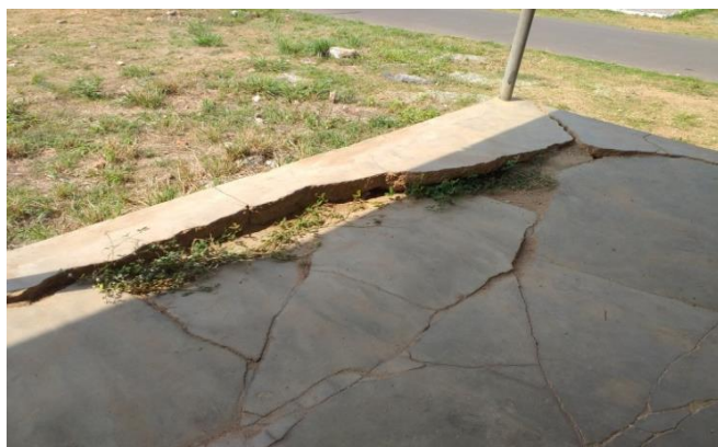
Plate 17: Dangerously Cracked Floor
