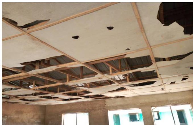
Plate 13: Asbestos Ceiling breakage
