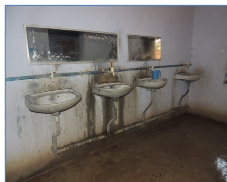
Figure 14: Poorly maintained toilets
