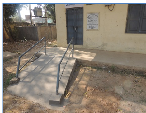
Figure 12: Ramp in Rayagada Auto. college, Rayagada
