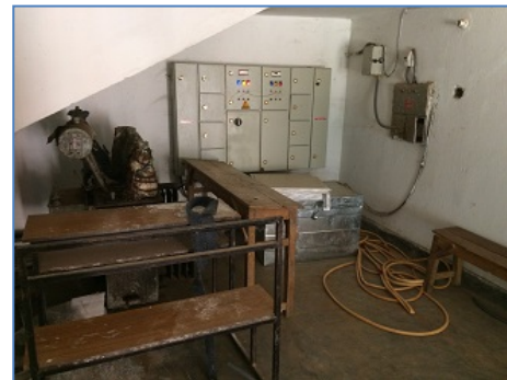
Figure 8: Unsafe electrical panel
