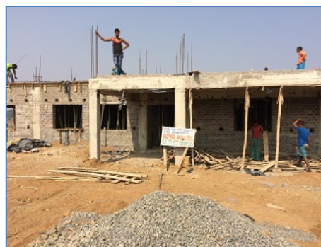
Figure 11: No safety measures at the construction site
