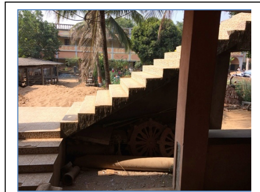
Figure 4: Unsafe staircase in a college
