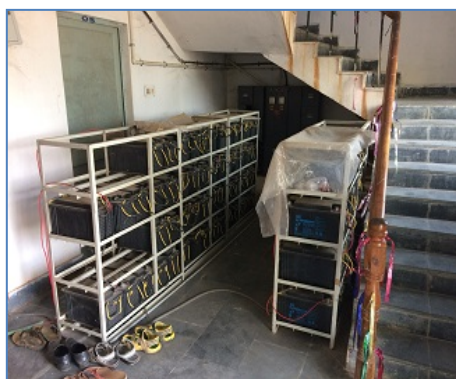
Figure 17: Batteries kept under the stairs
