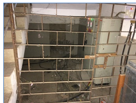
Figure 9: Protected electrical panel in Govt. Women's College, Baripada
