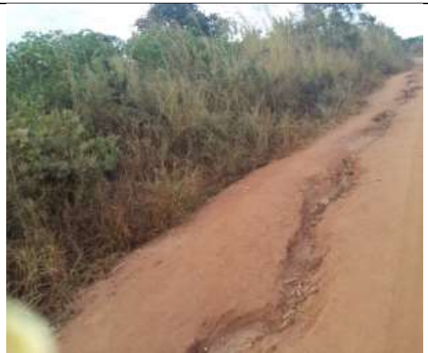
Picutre: Road from Zero to Murrumbala Sede
