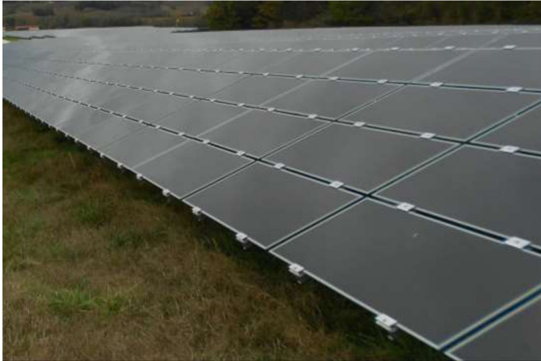
Figure 3.5: Typical appearance of Thin-Film CdTe Arrays
