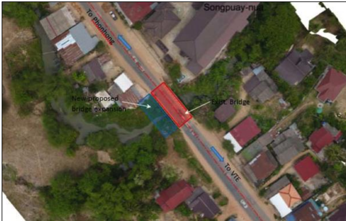
Figure 3-19: Proposed Bridge Expansion Location, Nam Houm
