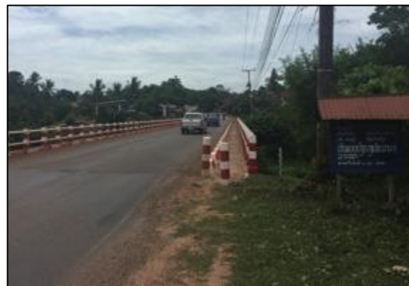
Figure 3-12: Bridge 7: Nam Cheng
