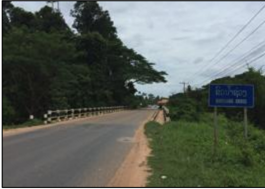
Figure 3-9: Bridge 4 – Nam Souang
