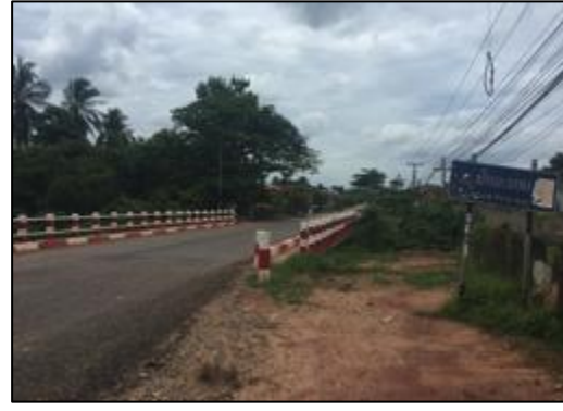
Figure 3-10: Bridge 5 – Nam Panai
