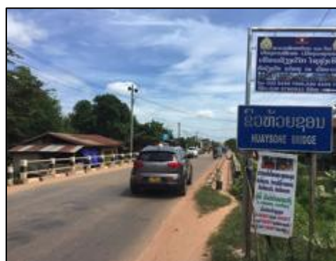
Figure 3-8: Bridge 2 - Houay Xone
