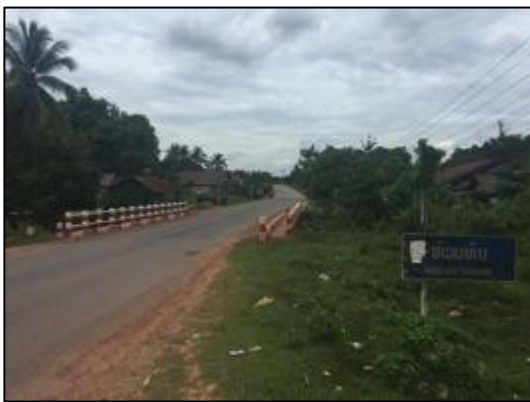
Figure 3-11: Bridge 6 – Houay Thonh
