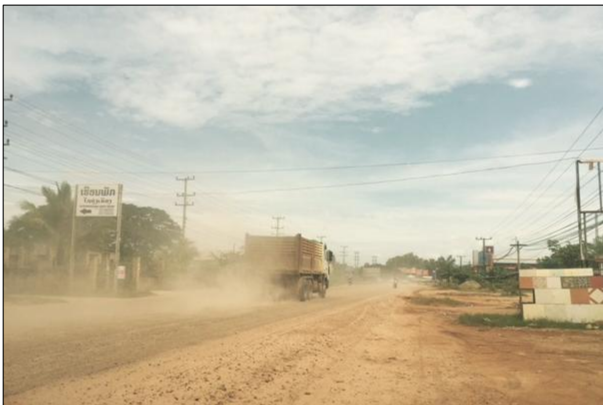
Figure 4-6: Unpaved Section of Road – KM3, June 2017
