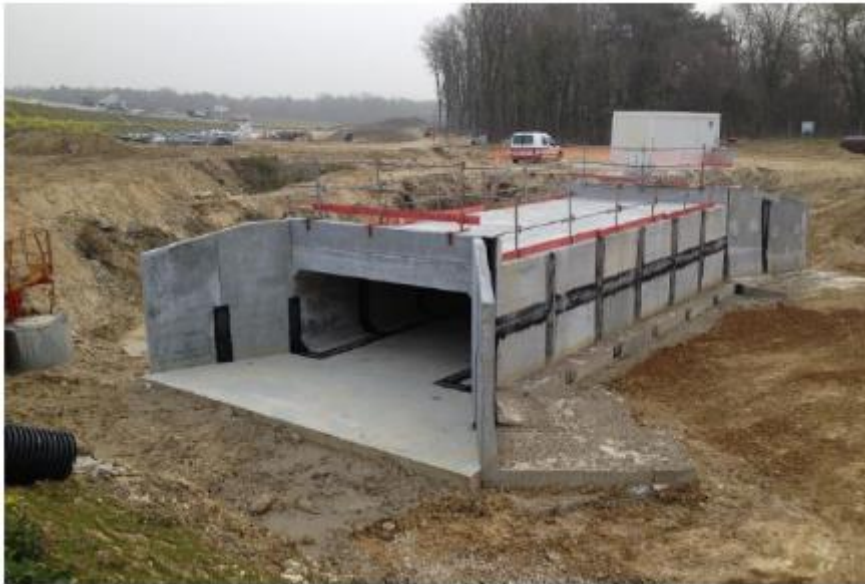
Figure 4-30 Example of a major Prefabricated Box Culvert
