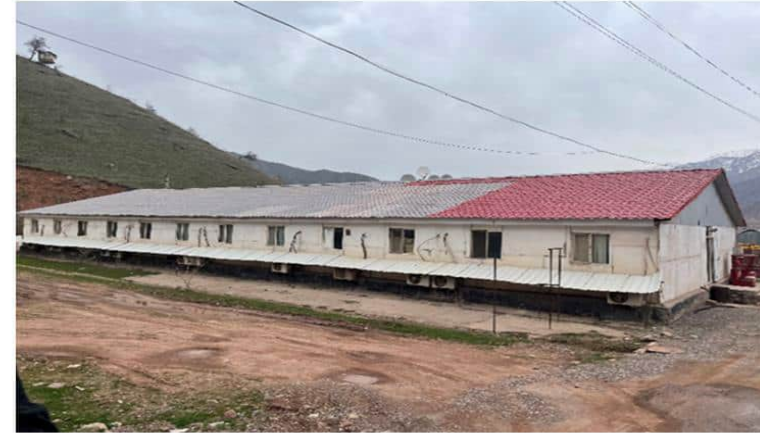
External View of Worker Accommodation Camp - Tunnel Sadd Ariana
