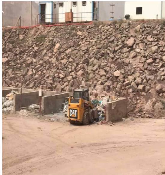
WeBuild General waste storage area
