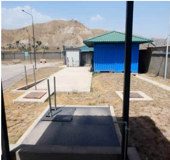
WeBuild Accommodation Camp WWTP
