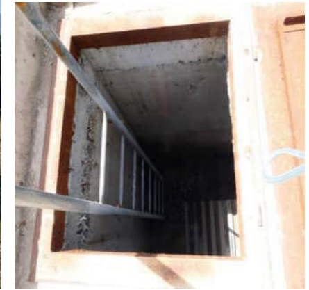
WeBuild WWTP holding tank
