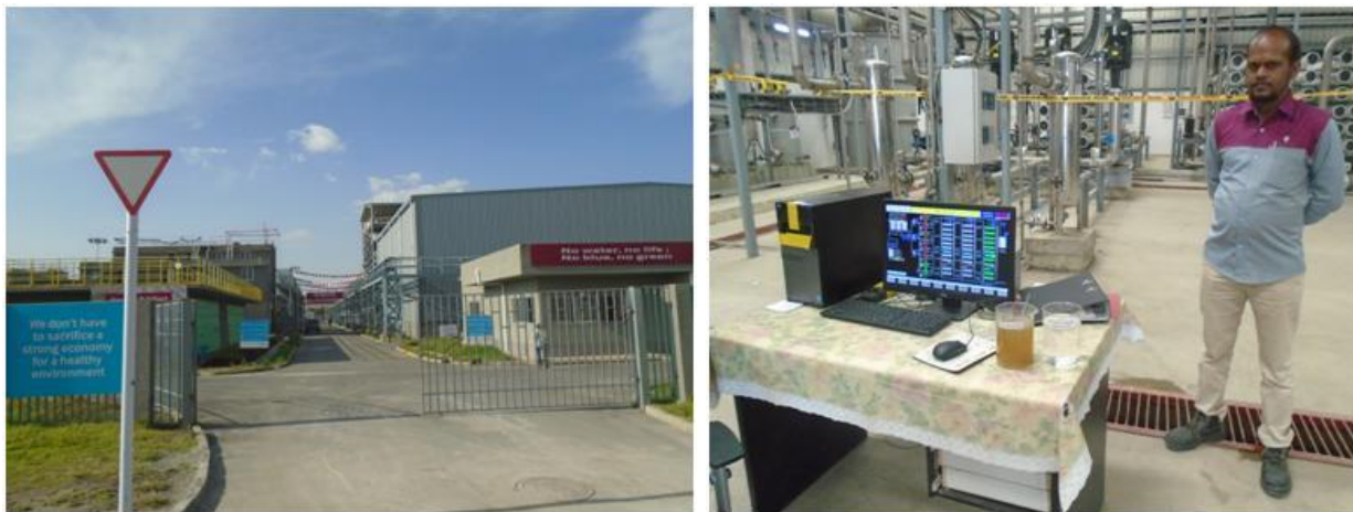
Figure 6. Partial View of Hawassa Zero Liquid Discharge WTP (left) and Showing Effluent Before and After Treatment in the WTP (right) (Source: WB Consultant 2017)
