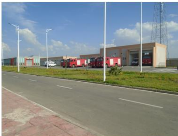
Figure 7. Partial View of the Fire Brigade Station and Clinic in Hawassa Industrial Park (Source: WB
