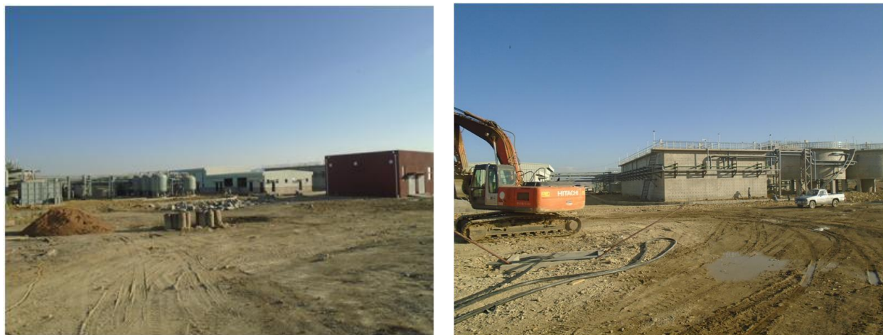
Figure8. Partial View of the Zero Liquid Discharge WTP Under Construction in Mekelle Industrial Park
