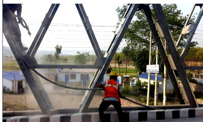
Sand Blasting work at Girwari Khola Bridge(45-H001-249)
