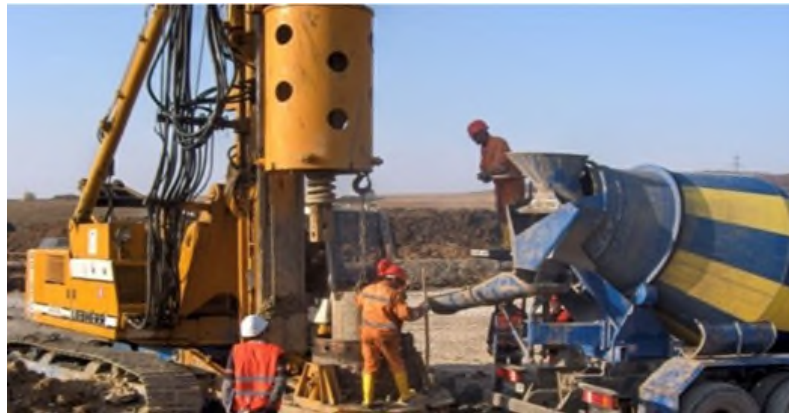
Figure 3-50. Pile Casting
