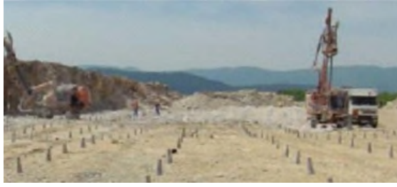
Location ready for filling with explosives.
