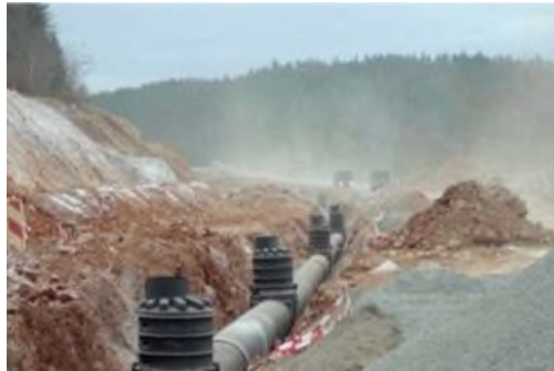
Collector pipe installation.
