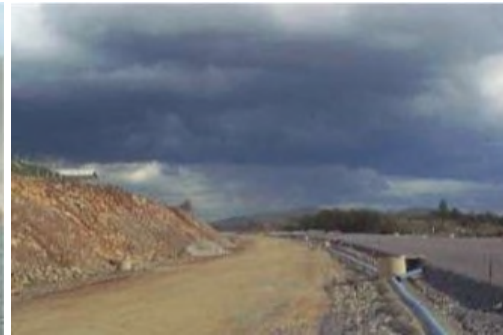
Perforated pipe installation.
