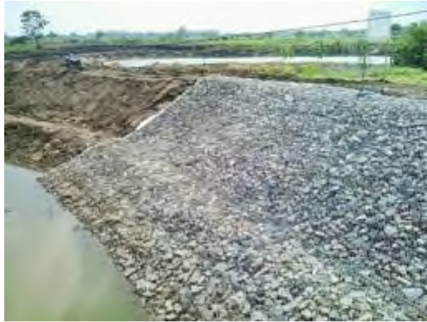
Figure 3-39. Example of Reno Mattress
