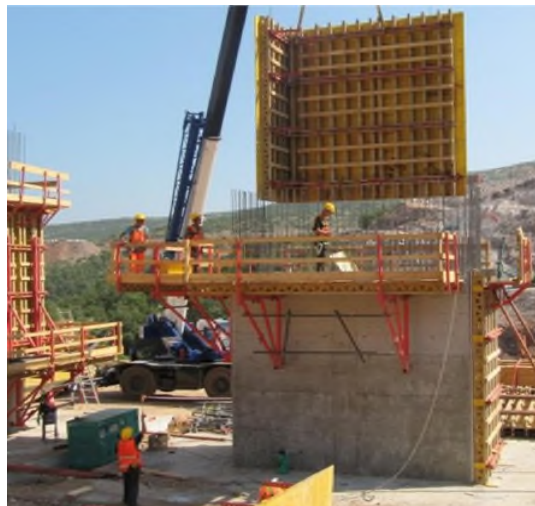
Figure 3-54. Pier Concreting
