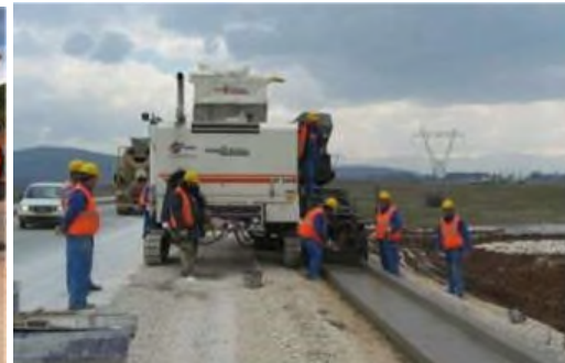
Channel and gutter operation - median and shoulder.
