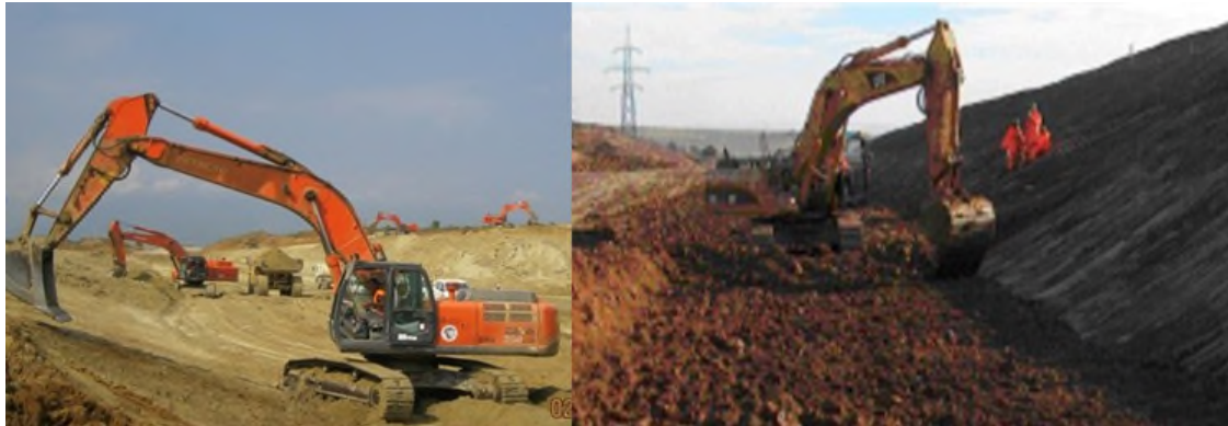
Excavation of common material with excavator.
