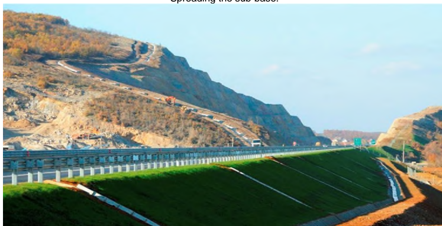
Concrete ditches and down chute construction.
