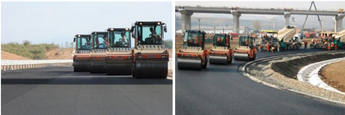
Figure 3-60. Drumrollers Compact the Asphalt Layer
