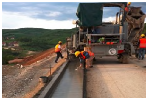
Channel and gutter operation - median and shoulder.
