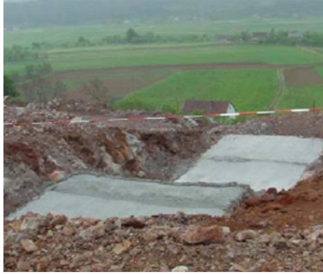
Figure 3-51. Lean Concrete Placement for Stepped Structural Foundation
