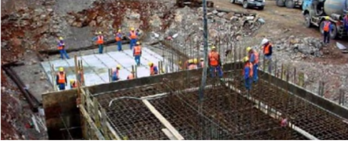
Figure 3-52. Foundation Concreting Operation
