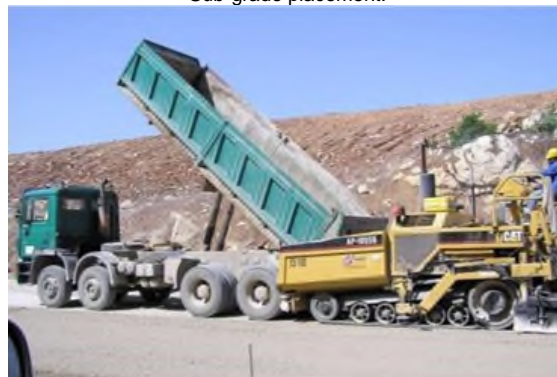
Spreading the sub-base.
