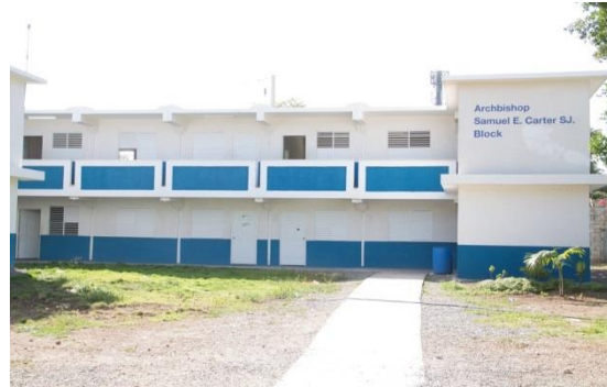
Reinforced Concrete Modular Structure
