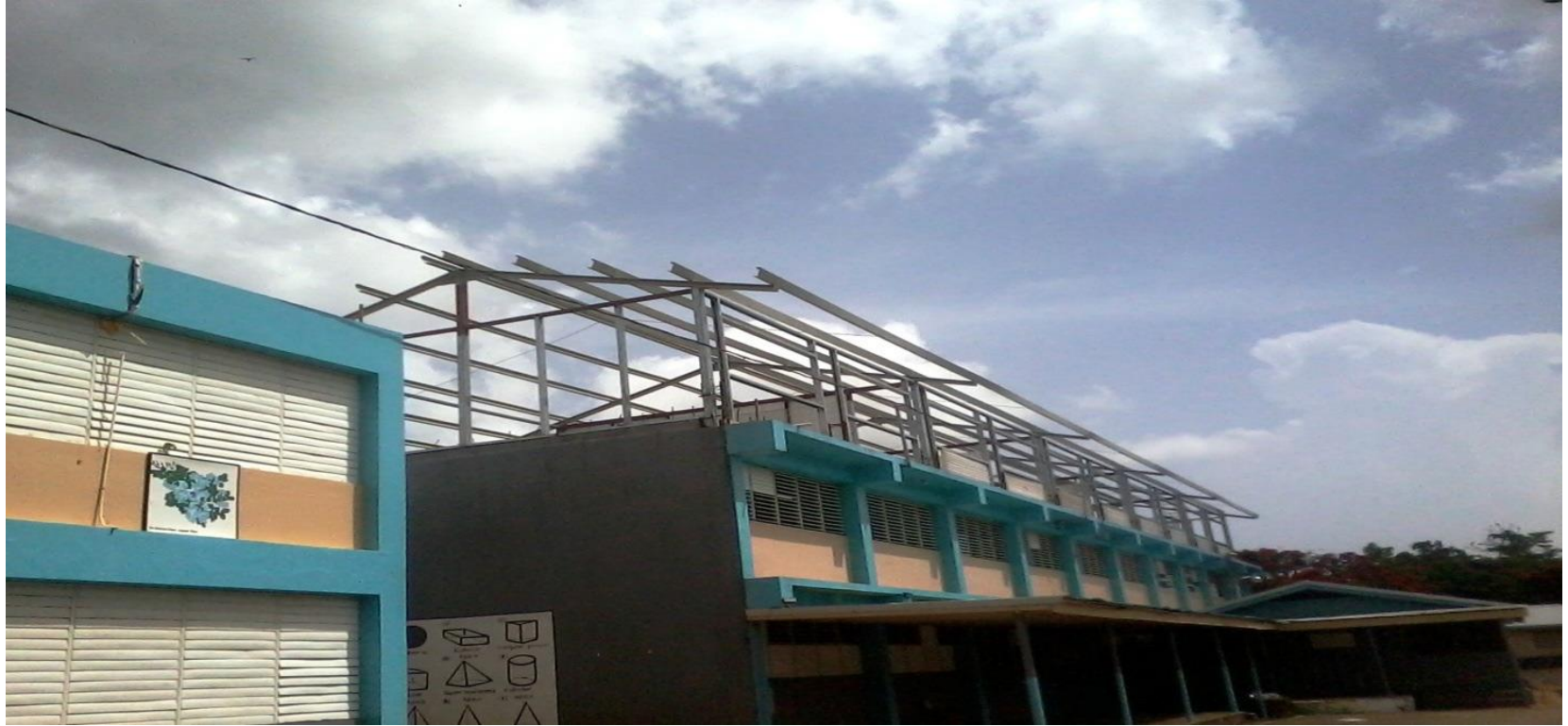
CONSTRUCTION OF A STEEL FRAME CLASSROOMS
