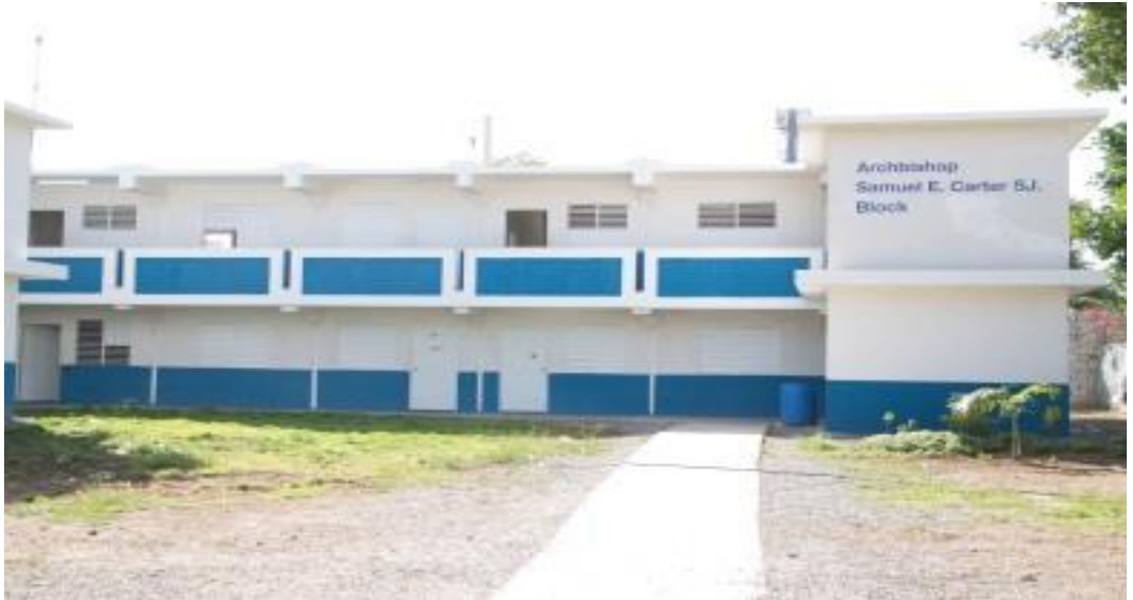
Two (2) Storey Reinforced Concrete Modular Classroom Block (Expansion Project)
