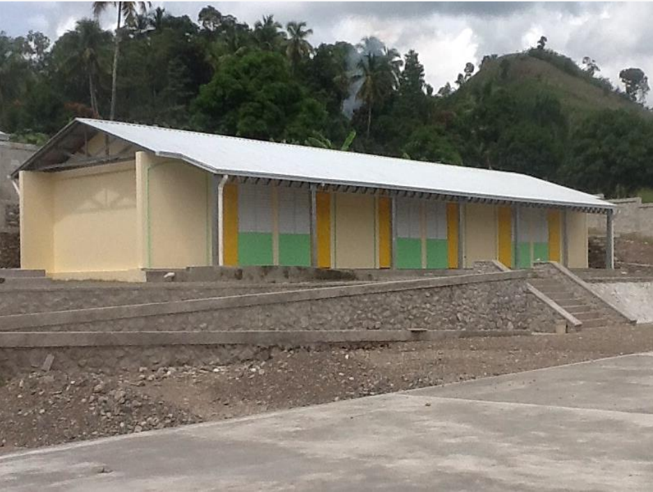
Confined masonry
