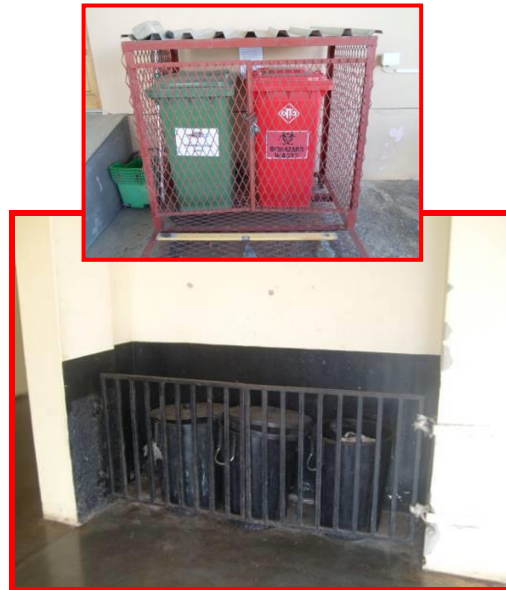
Figure 10-1 Temporary storage for waste
