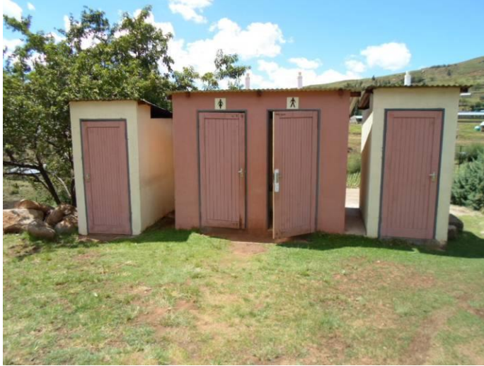
Figure A.3-16 Pit latrines at a Minor Health facility
