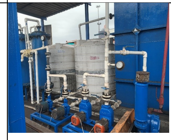
Photo 24. Sewage Treatment Plant 5 KLD
