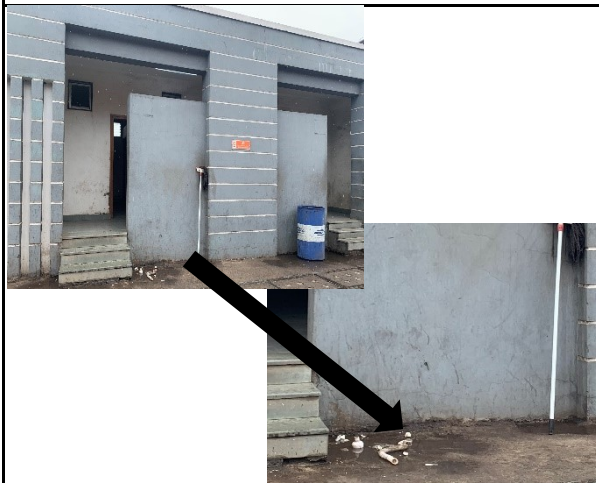
Photo 11. Electric Waste observed near Toilet
