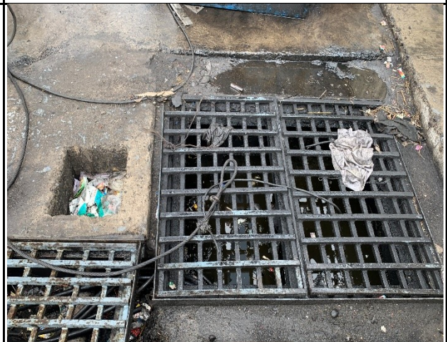
Photo 12. Plastic waste observed in Oil Separator Pit
