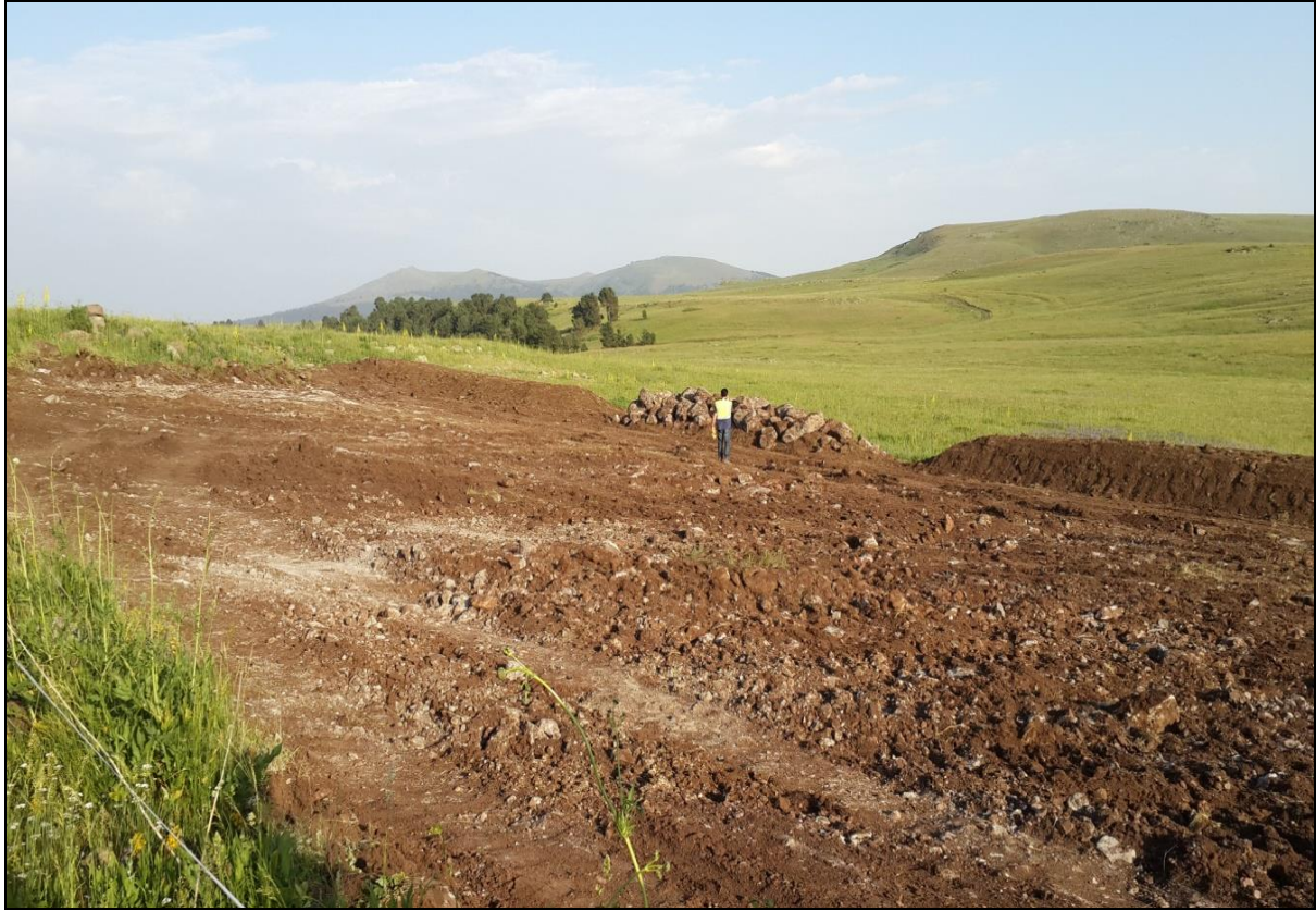
Picture 5.6.6.4. Topsoil Stripping Works in Stony Areas, Photo B. ERDEM, 2015
