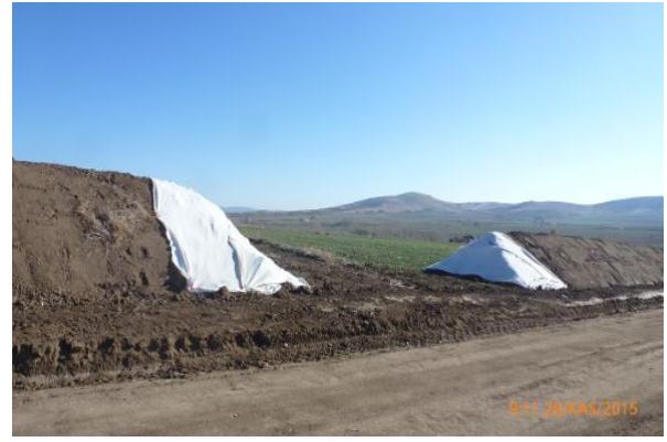
Picture 5.6.6.8. Gaps left between the stockpiles in the topsoil storage areas, Photos: B. ERDEM, 2015
