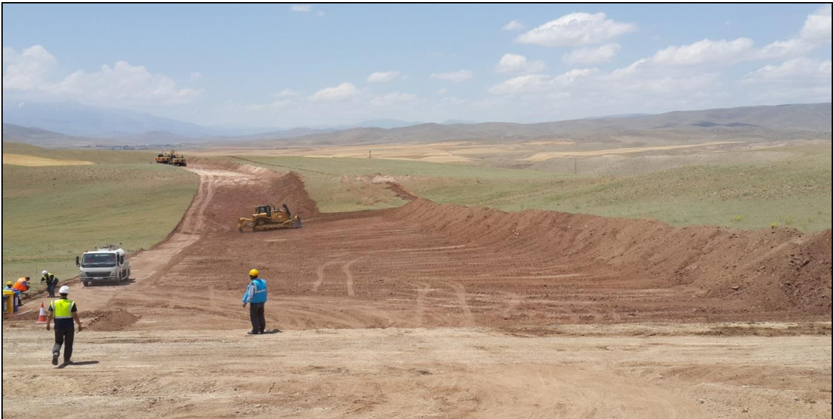
Picture 5.6.6.3. Topsoil Stripping Works during Construction Period, Photo: B. ERDEM
