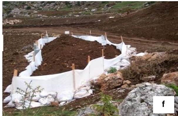
Picture 5.6.6.5. continued In the scope of topsoil storage methods a-Stone support, b,c-Geotextile sheeting, and d,e,f-silt fence applications, Photos B. ERDEM, 2006
