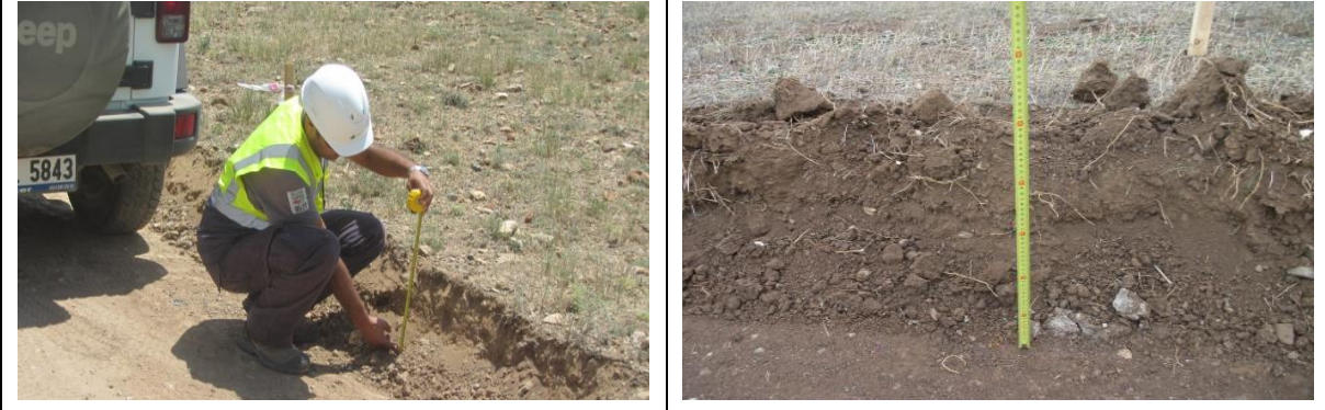
Picture 5.6.6.2. Topsoil Stripping Works, Control of Stripping Depth, Photo: B. ERDEM , 2015
