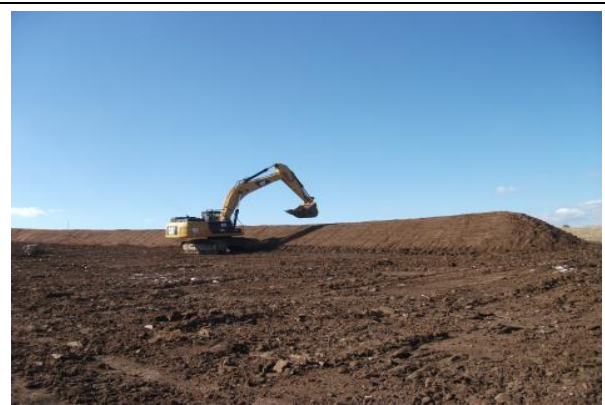
Picture 5.6.6.10. Works for Compaction of Stockpiles in Topsoil Storage Areas, Photos: B. ERDEM, 2015
