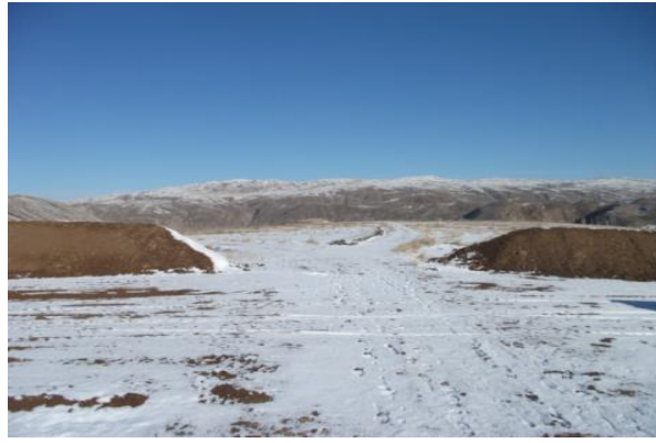
Picture 5.6.6.8. Gaps left between the stockpiles in the topsoil storage areas, Photos: B. ERDEM, 2015
