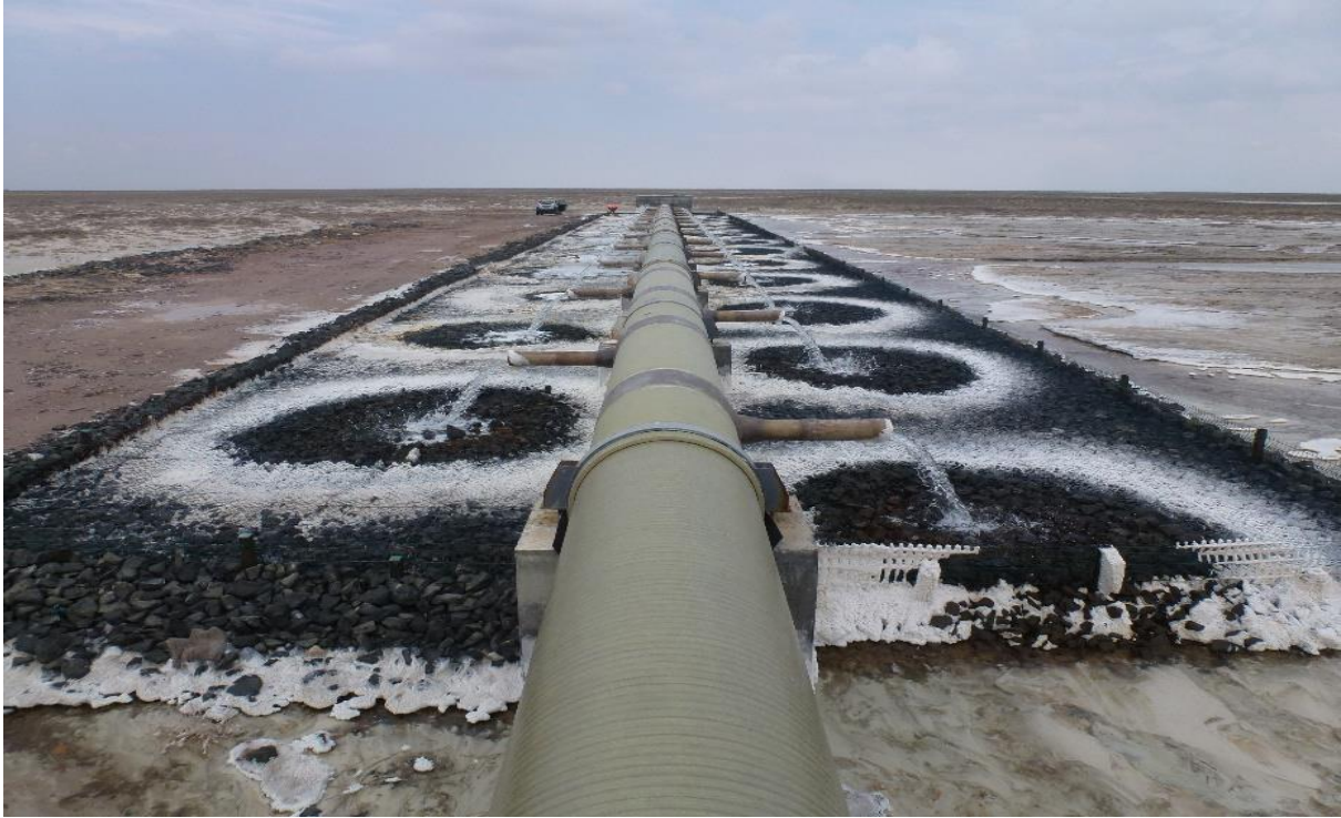
Picture 3.3.1.1. A view from Brine Discharge Point of Underground Gas Storage Project where Leaching Process is in Progress
