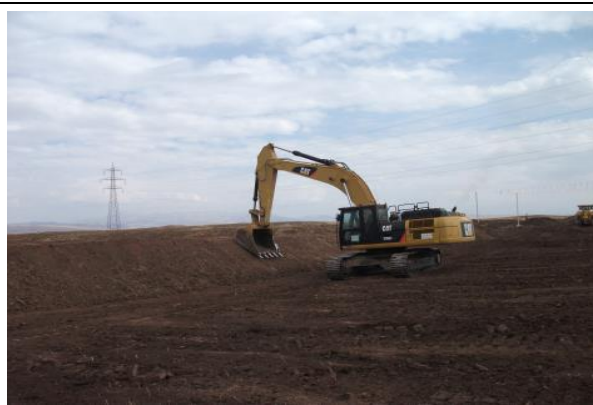
Picture 5.6.6.10. Works for Compaction of Stockpiles in Topsoil Storage Areas, Photos: B. ERDEM, 2015
