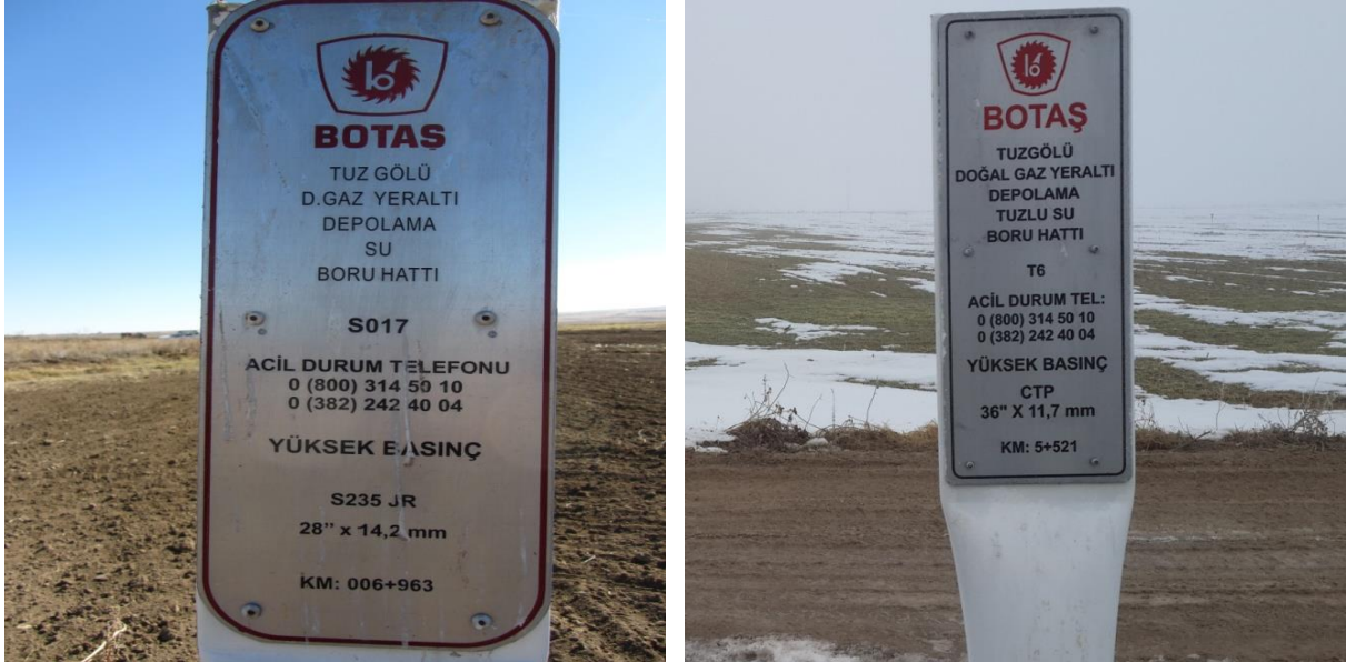
Picture 3.4.1.2. Views of Line Markers Used on the Routes of Fresh Water line and Brine Discharge Line under the Underground Gas Storage Project (December 2015)
