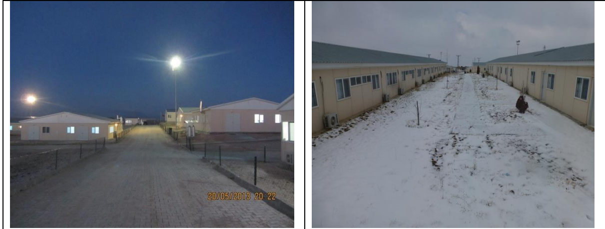
Picture 3.3.1. A view from campsite on Underground Gas Storage Project Under Construction
