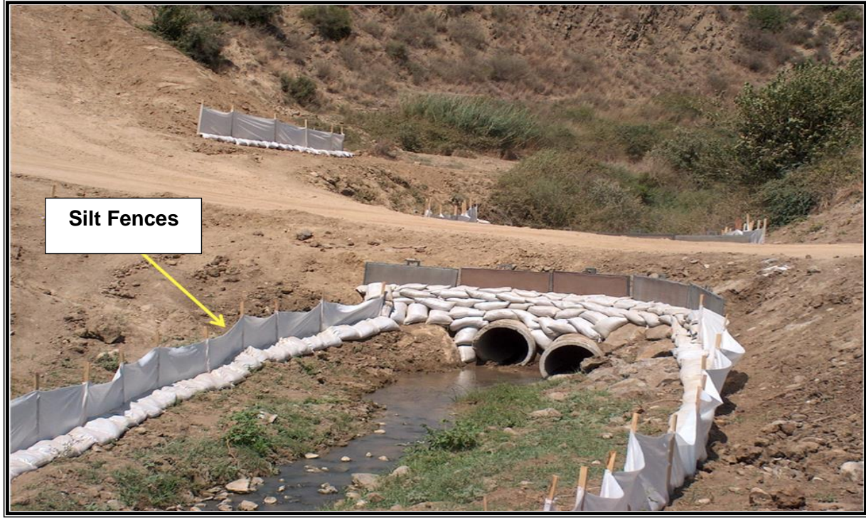
Picture 5.6.6.12. Silt Fence Application for Sedimentation Control, Photo B. ERDEM, 2005
