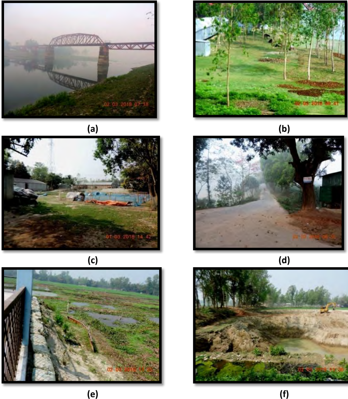
Figure 3.17: Selected sites (preliminary) for construction of various components of BMWSSP's sub-project at Ullahpara of Sirajganj District: (a) Raw water Intake site, Karotoya River (b) Booster pump station (c) Proposed location for water treatment plant (d) Proposed Water distribution pipelines along the road (e) Overhead tank site in the low-land and (f) Agro-wetland for de-sludge unit / waste dumping unit.
