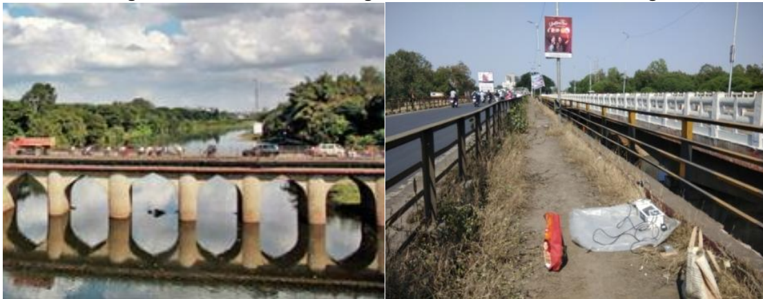
Figure 4.9: Vibration Monitoring Location and Results at Harris Bridge
