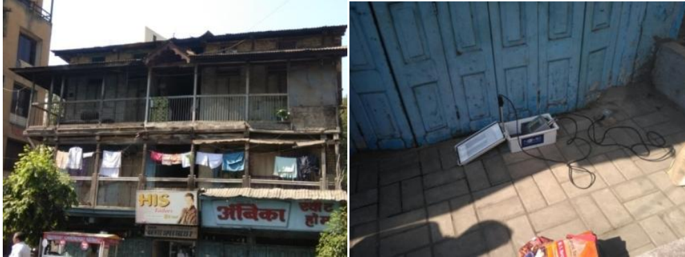
Figure 4.16: Vibration Monitoring Location and Results at Old Wooden Structure at Mandai
