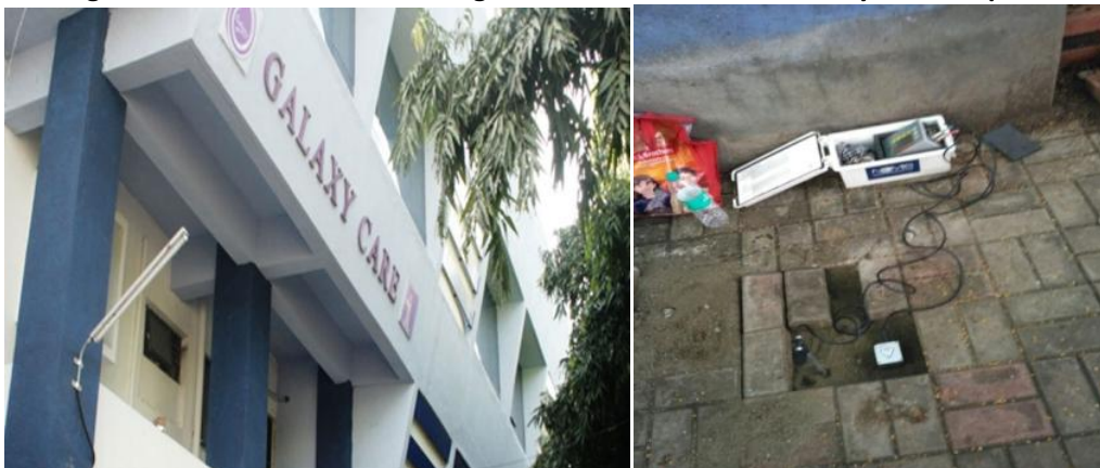
Figure 4.18: Vibration Monitoring Location and Results at Galaxy Care Hospital
