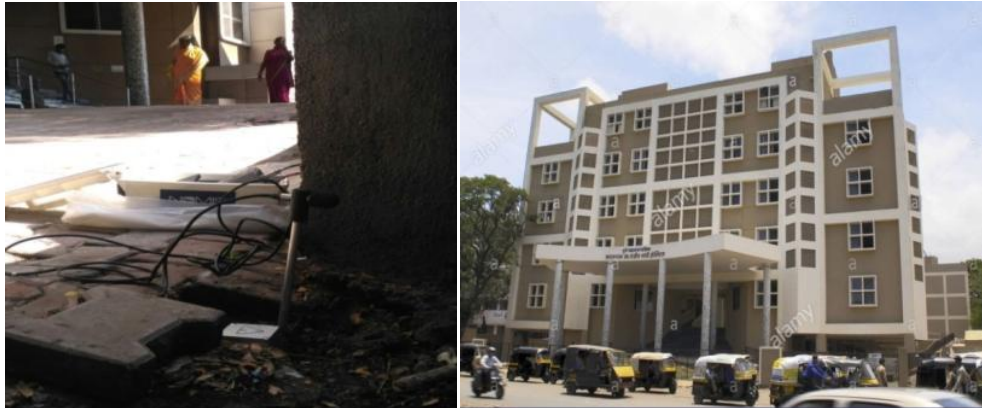
Figure 4.22: Vibration Monitoring Location and Results at Rajiv Gandhi Hospital
