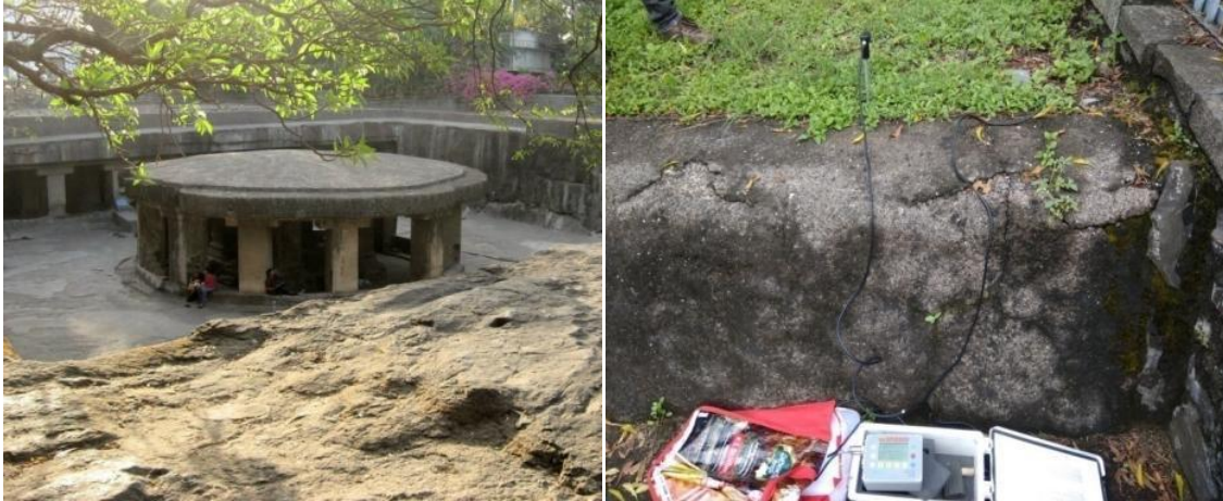
Figure 4.10: Vibration Monitoring Location and Results at Pataleshwar Cave Temple
