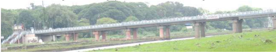
Figure 7.11: Photograph of a Reinforced Concrete Bridge
