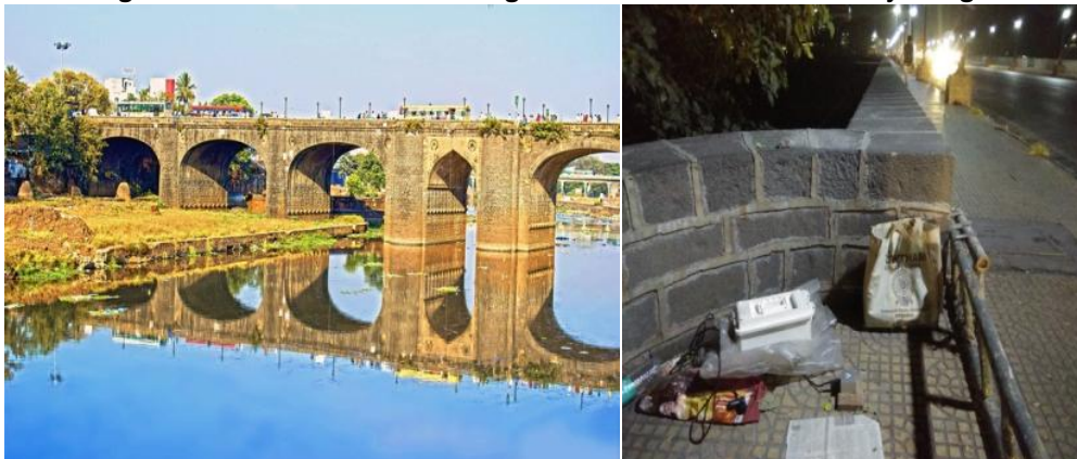
Figure 4.19: Vibration Monitoring Location and Results at Shivaji Bridge
