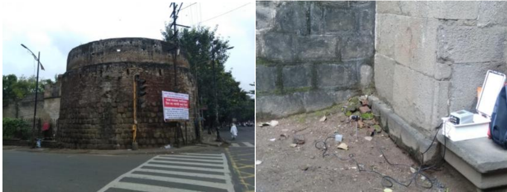
Figure 4.12: Vibration Monitoring Location and Results at Shaniwar Wada
