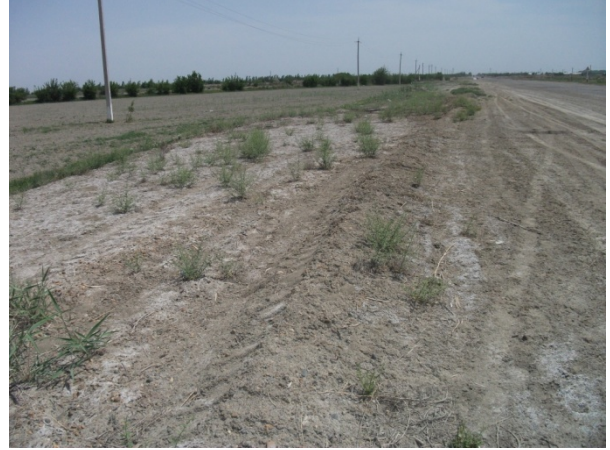
Salted lands along the project road (km 249)
