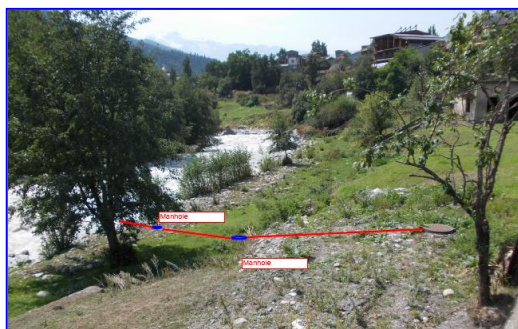
Fig. 12: Route of outfall collector (1) and nearest users downstream
