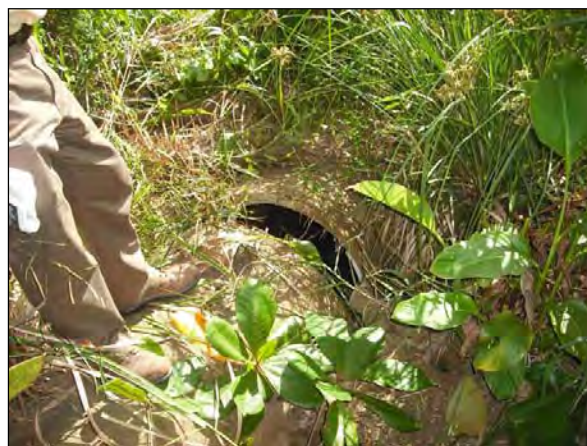
Figure 3-5 Section of Trunk Sewer along Vistabella River Showing Open Joint
