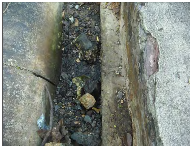
Figure 3-4 Section of Trunk Sewer Along the Sea Wall Showing Possible Points of Inflow at Pipe Joints
