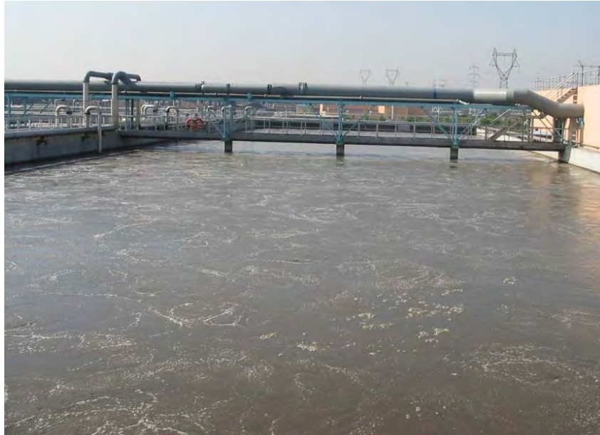
Figure 3-17 Fine Bubble Aeration Bioreactor
