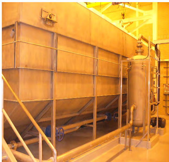
Figure 3-21 Stainless Steel DAF Tank
