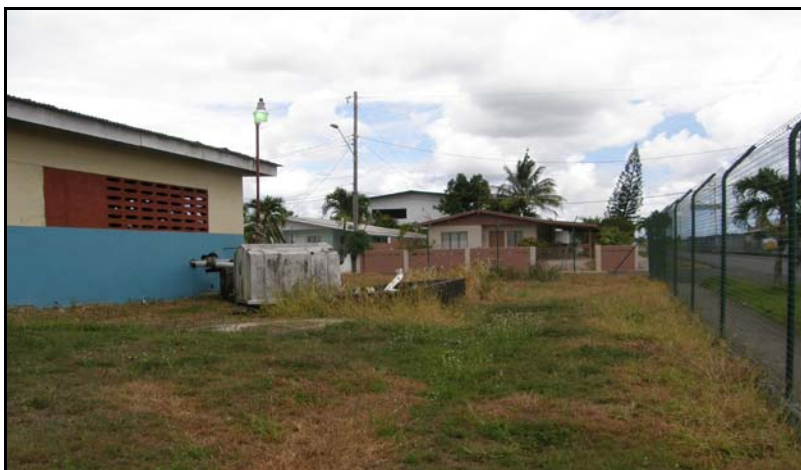
Photograph 3.7: Malabar Lift Station
