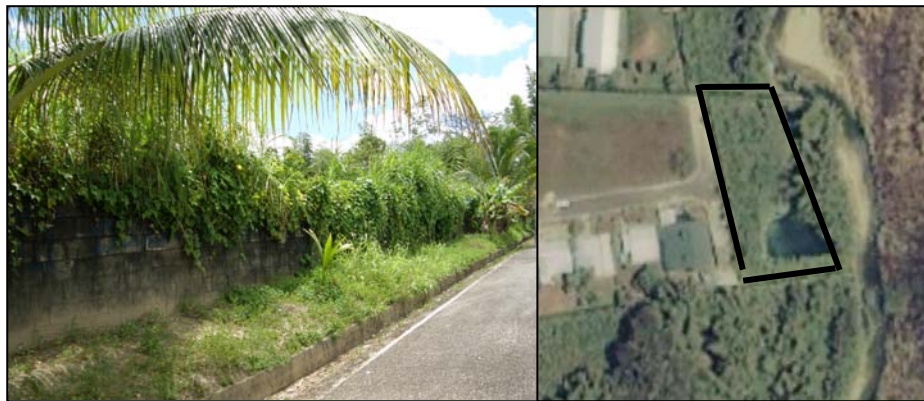
Photograph 3.3: Tumpuna Gardens Wastewater Treatment Lagoons
