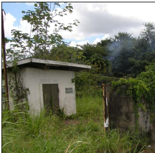
Photo 3.8: Santa Rosa Springs Lift Station
