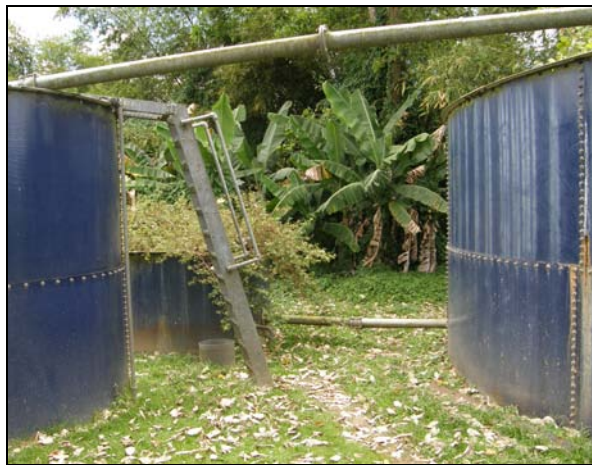
Photograph 3.1: Hermitage Heights WWTP
