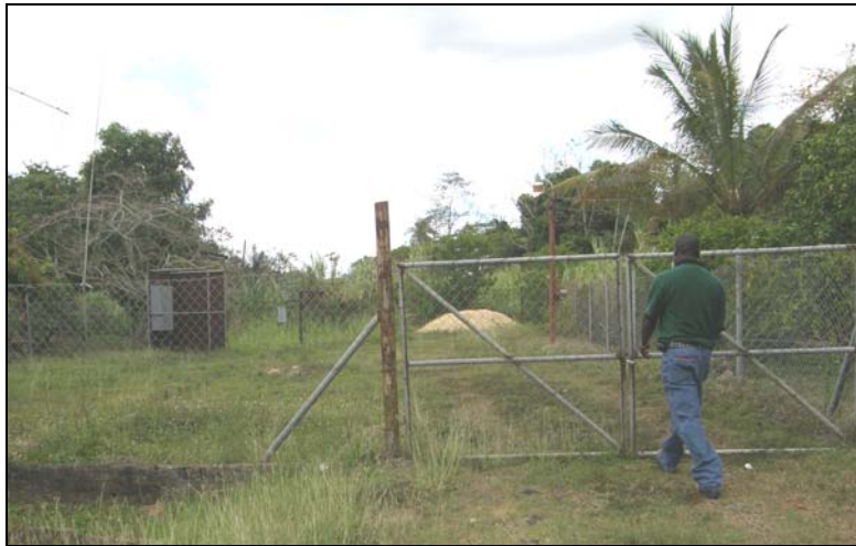
Photograph 3.4: Carib Homes Lift Station
