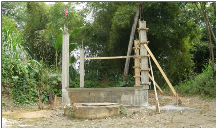
Photograph 3.6: Dundee Lift Station
