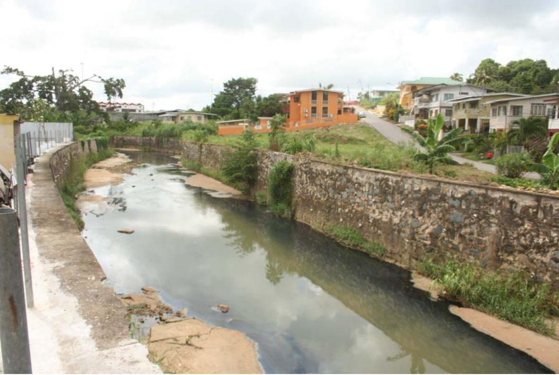
Plate 1 Ciperó River in concrete channel at grid reference 668521, 1134820
