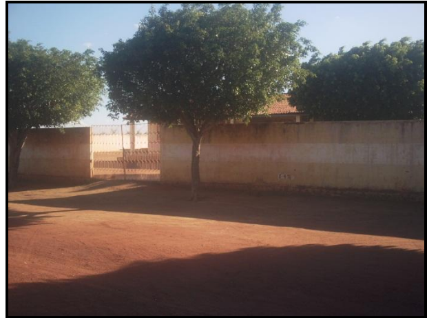
Escola as margens do trecho CE-187 Salitre - Divisa CE/PE
