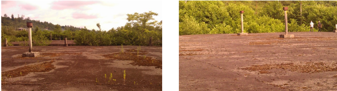
Fig. 1 Existing Bashi Reservoirs
