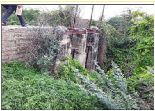
Plate 13 : Debris around Head Regulator
