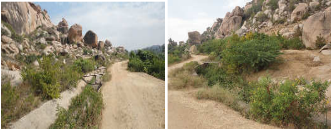
Figure 17: Location along Anegundi Canal where stormwater runoff directly enters the canals
