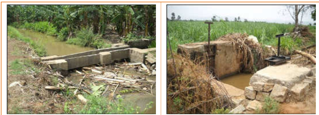
Plate 3: Channel used as a disposal point
