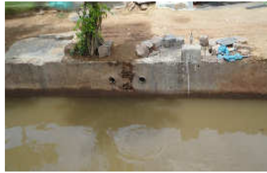
Town sewage directly draining into Basavanna Canal within Hospet Town limits
