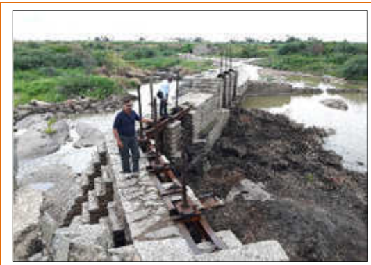
Plate 13 : Debris around Head Regulator
