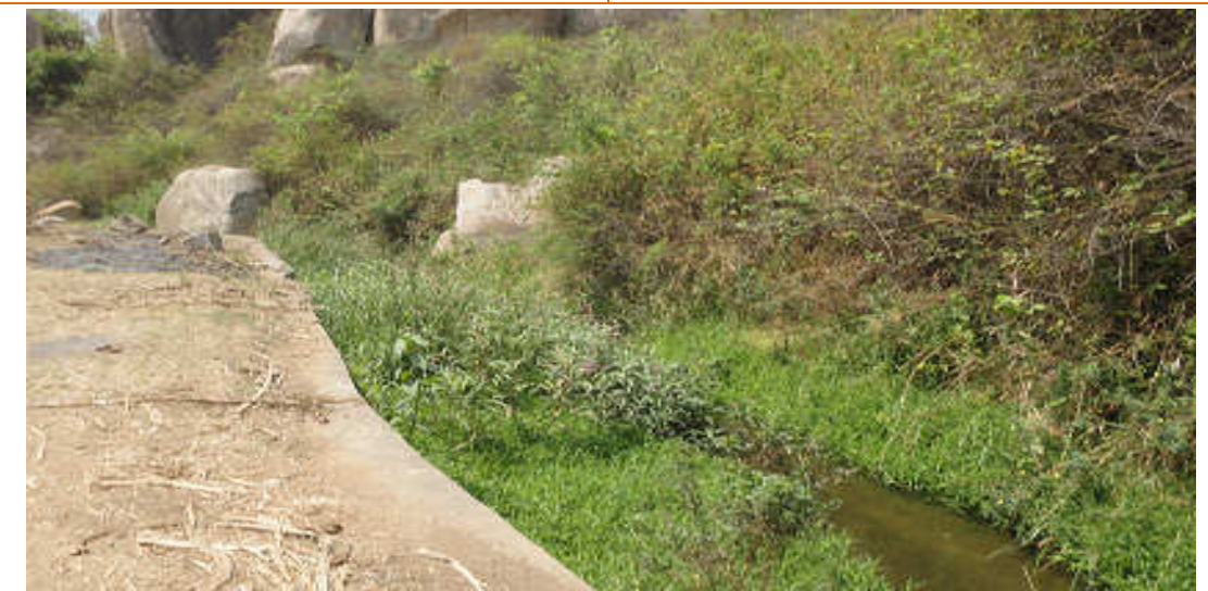
Thick vegetative growth in Aneundi Channel hampering flow of water
