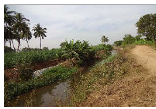
Plate 14: Breach in channel section
