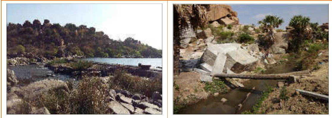
Plate 1: Deteriorating anicuts and other structures requiring immediate rehabilitation
