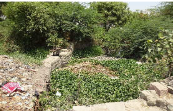
Siruguppa Canal within Siruguppa Town used as part of Town Sewerage System
