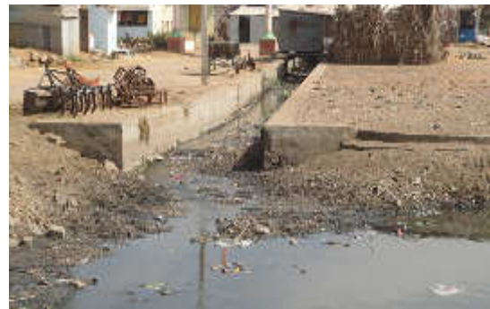
Municipality sewage in some stretches of Kampli Canal
