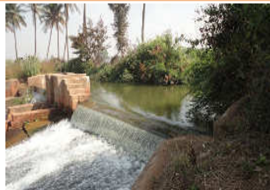
A structure on Raya Channel in need of rehabilitation
