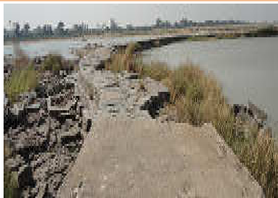
A typical damaged VNC anicut
