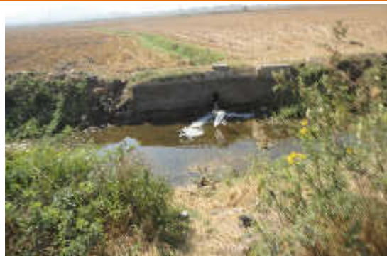
Degraded banks of the Siruguppa Channel
