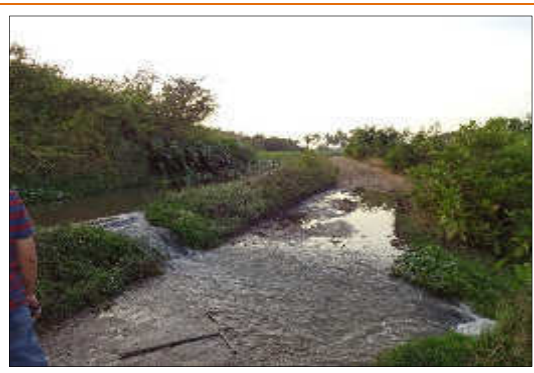
Plate 14: Breach in channel section
