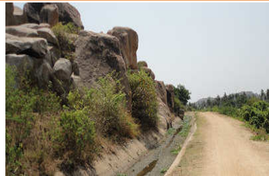
Silting in Aneundi Channel
