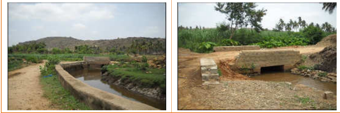
Plate 4: Channel reaches with size stone masonry lining
