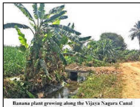
Banana plant growing along the Vijaya Naguru Canal
