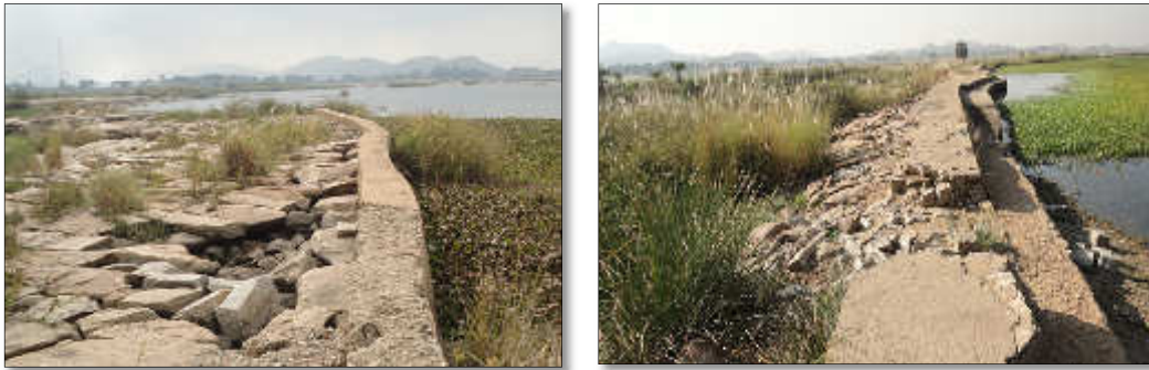
Figure 20: Typical Work within the OCR Area: Need for Realigning and Strengthening of Anicuts to prevent seepage
