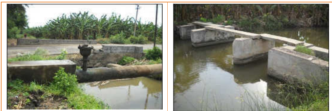
Plate 7: Damaged service road
