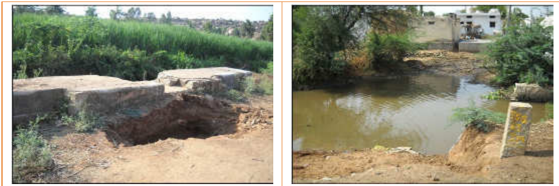
Plate 5: Damage due to seepage and poor maintenance
