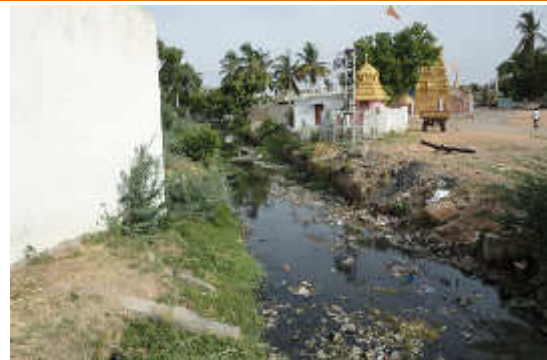
Solid waste dumping and sewage ingress into Upper Gangavathi Canal in Gangavathi Town
