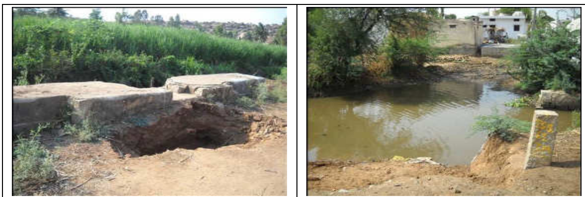
Plate 5: Damage due to seepage and poor maintenance
