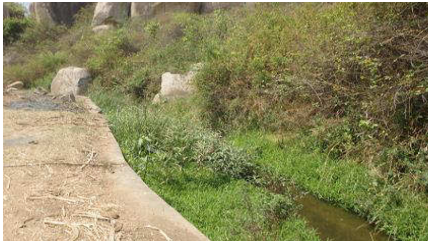
Thick vegetative growth in Anegundi Channel hampering flow of water
