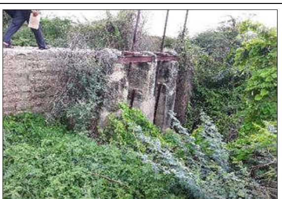
Plate 13 : Debris around Head Regulator
