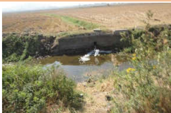
Degraded banks of the Siruguppa Channel
