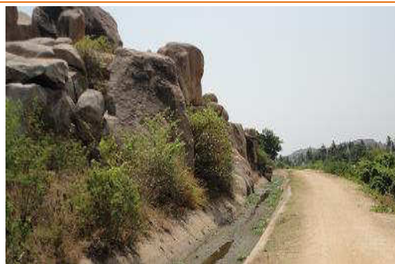
Silting in Anegundi Channel
