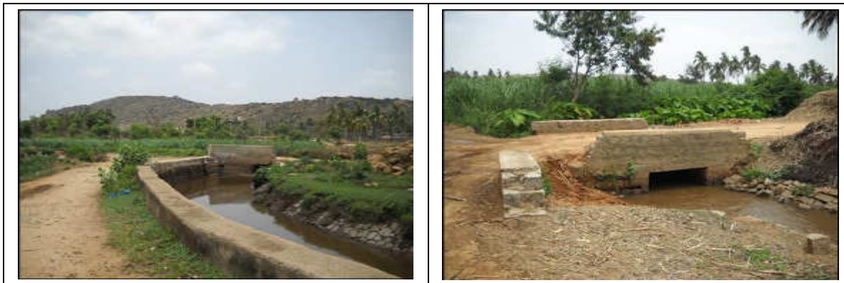
Plate 4: Channel reaches with size stone masonry lining
