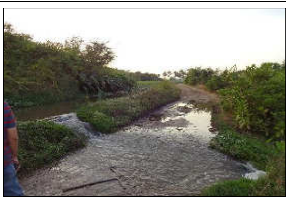
Plate 14: Breach in channel section
