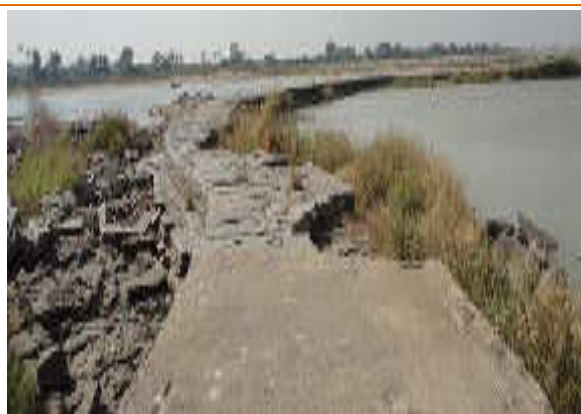
A typical damaged VNC anicut
