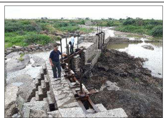
Plate 13 : Debris around Head Regulator
