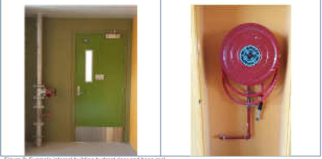
Figure 2: Example internal building hydrant riser and hose reel.
