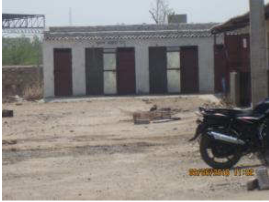
Gender specific toilet and bathrooms at labour camp
