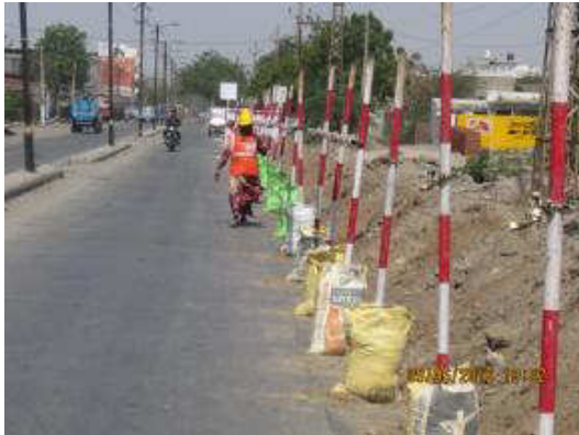
Barricades provided at site
