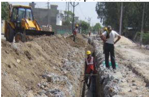
Use of PPEs by workers at site
