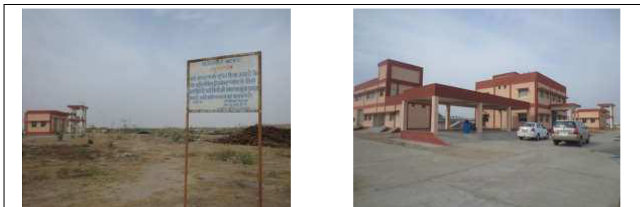
Existing STP and premises-Balance land is adequate for construction of new STP under RUIDP-III
