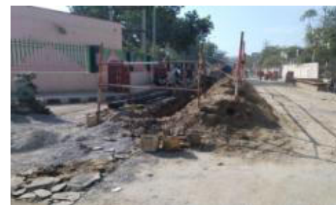
Barricades provided at Water Supply Pipe laying site
