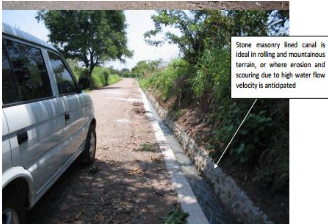
FMR with concrete/stone masonry lined canal. (ARCDP2)
