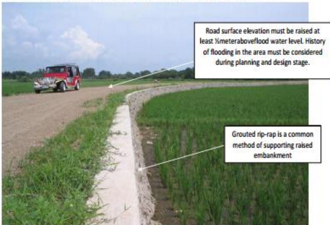
FMR with raised embankment supported by concrete stone masonry or grouted rip-rap retaining walls. (ARCDP2)
