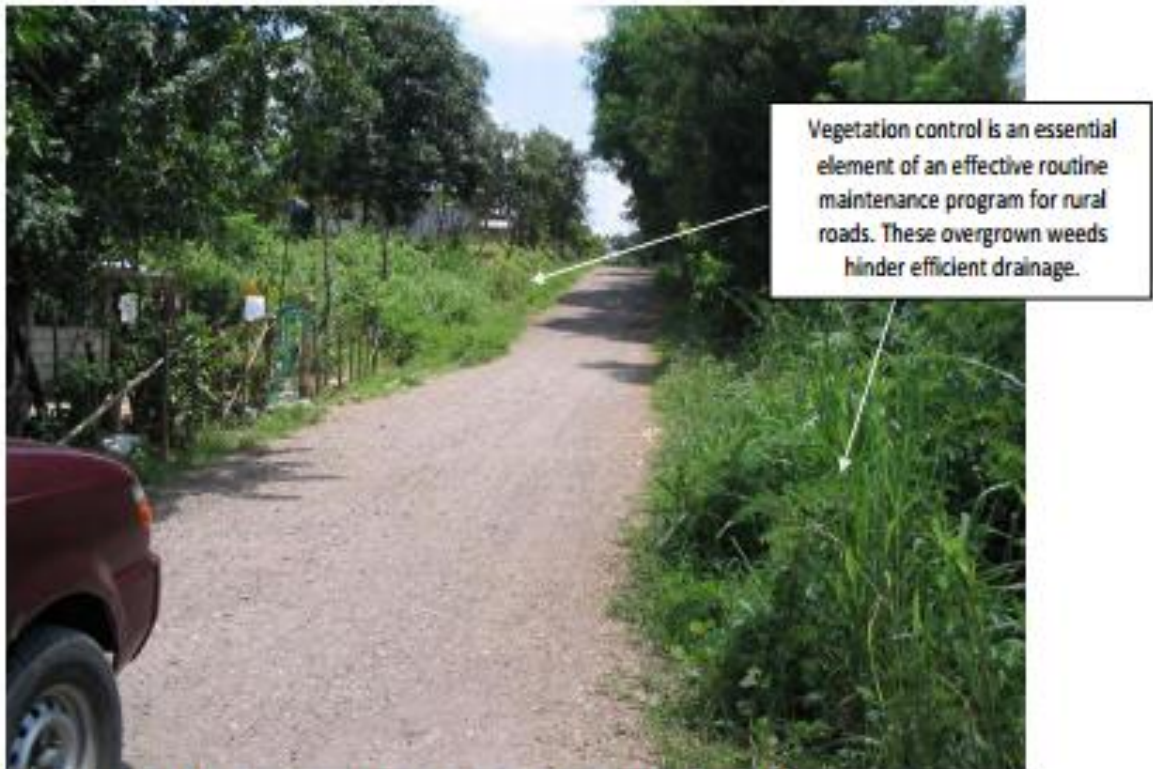
FMR with side ditches covered with over grown vegetation. (ARCDP2)
