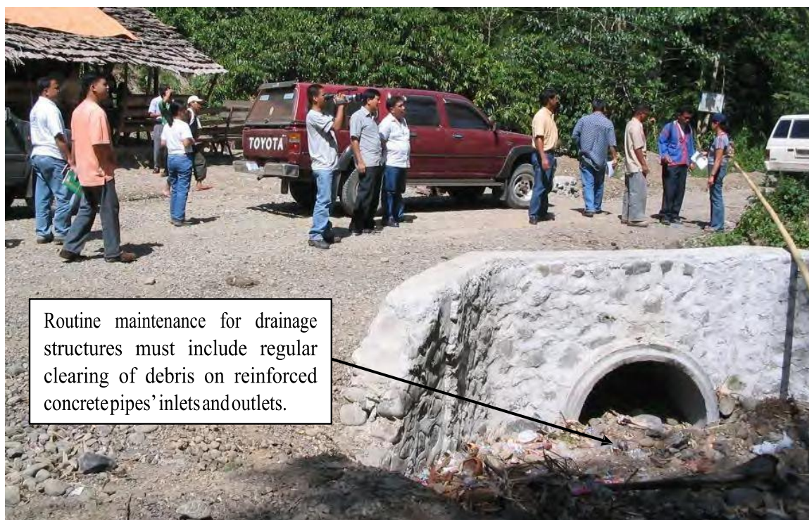
Cross drainage structure half-filled with debris. (MRDP1)
