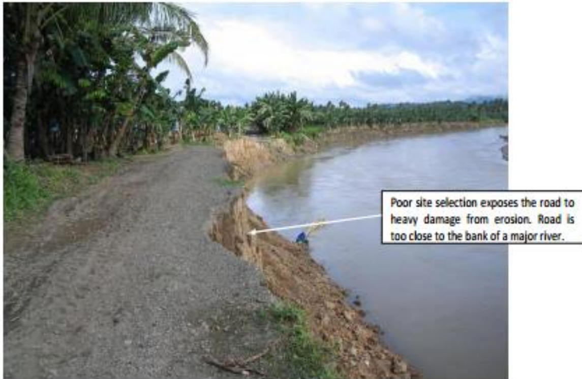
FMR damaged due to scouring
