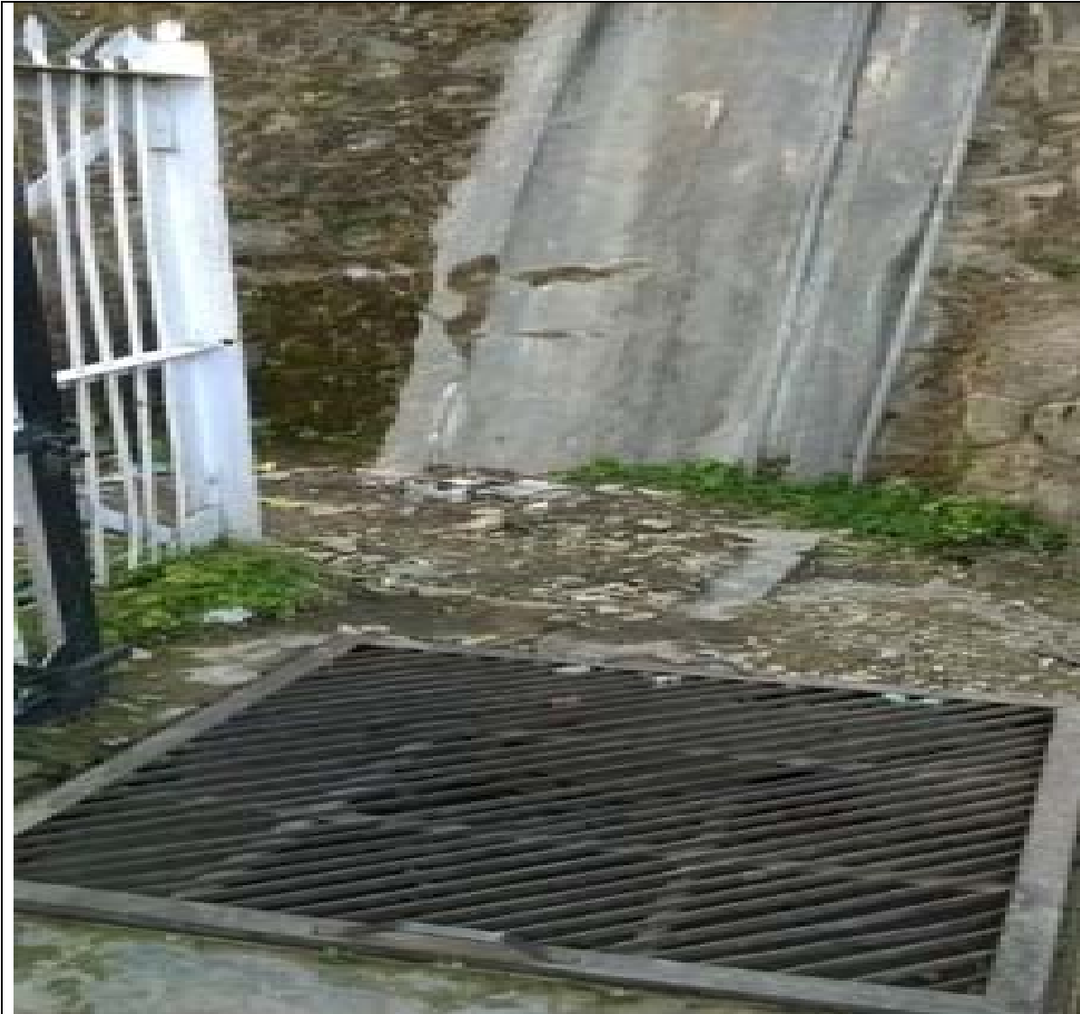
Chocked storm water drain in ITI Tehri
