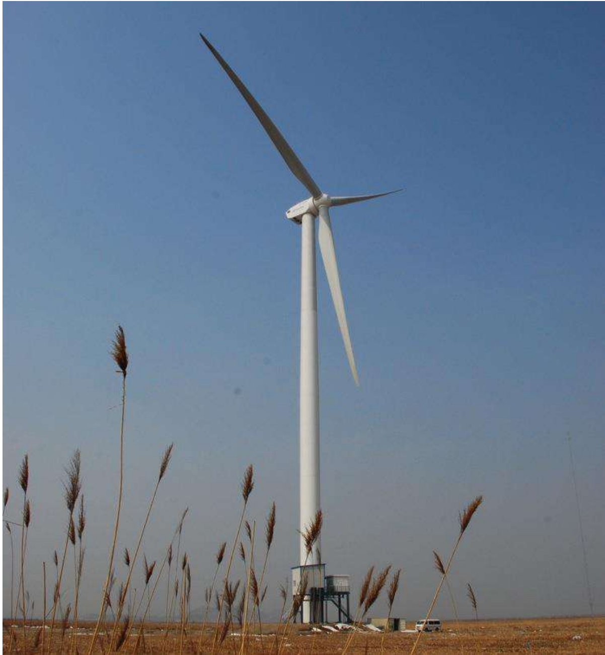
GW 2.5MW, Guanting Olympic Wind Farm
