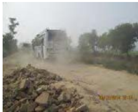
Broken pavement and dust emission at km 25.700
