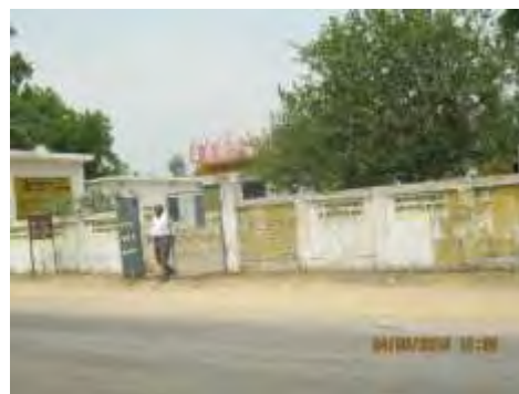
School along Mohanlalganj-Unnao
