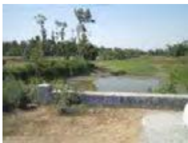
Fig. 52: Pond at km 17.400 in Village Chargharwa
