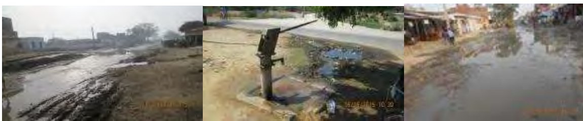
Fig 39: Water logged sections along the Project Roads
