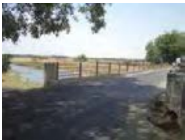
Fig. 56: Sai River at km 13.100 in Village Jabrella
