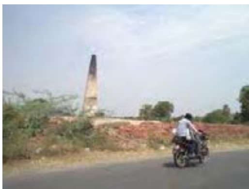
Brick kiln at km 15.400 in Pitna Kheda
