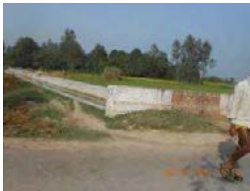
Fig.48: Canal at km 14.950 across the road in Luxmanpur
