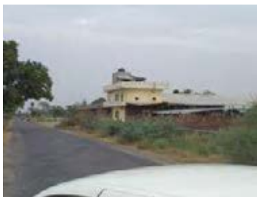
Pipe Industry at km 55.200 in Taura Bichia
