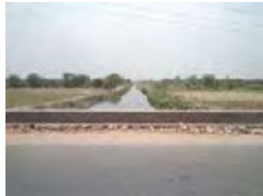
Fig. 57: Canal at km 1.100 in Mohanlaganj
