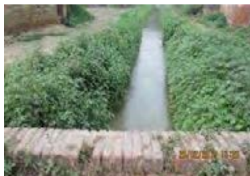
Fig.50: Canal at km 16.900 across the road in Delhi Bazaar
