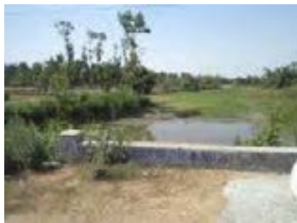
At km 17.400 (LHS) in Chargarwa- 15m from CL along Kaptanganj-Naurangia
