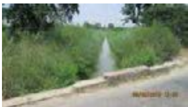
Fig.59: Canal at km 39.550 in Village Gadka
