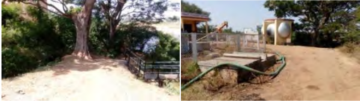
Proposed site for construction of Jack well and existing jack well site in Rajanahalli
